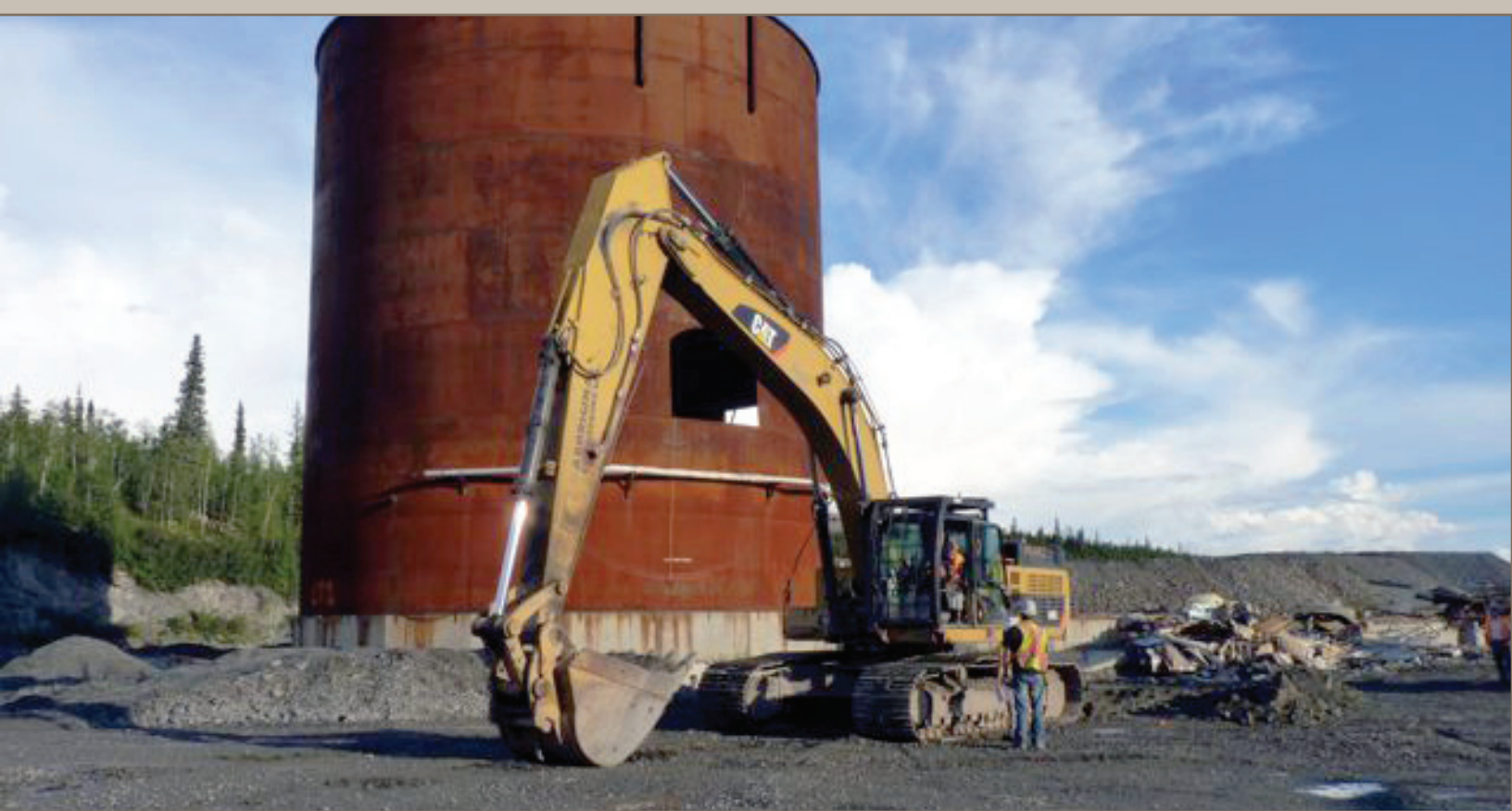
One of twelve leach tanks requiring decontamination
