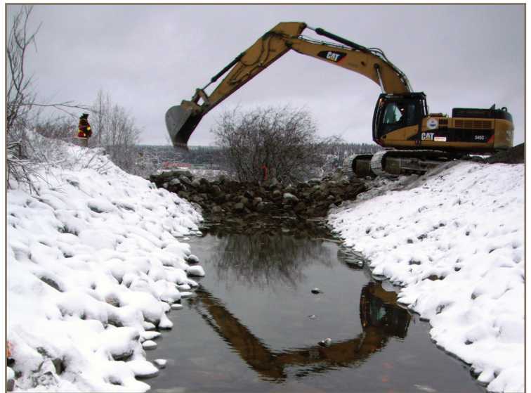
Installation of the dam in the Spot Pond to Truck Lake Drainage Channel
