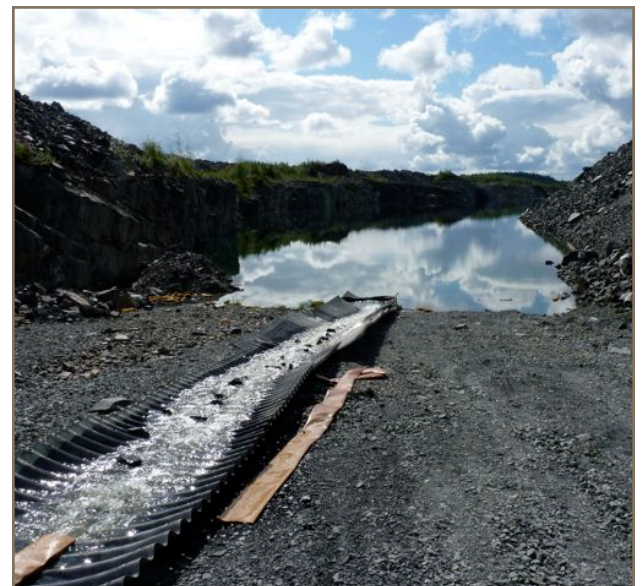
Corrugated steel pipe used to aerate discharging water in zone 2.0 pit
