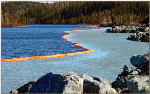
Effective containment of turbidity caused by construction activities
