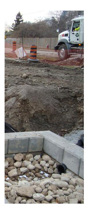
The Elm Drive retrofit pilot project involved a nonstandard road design, as well as the implementation of bioretention planters within a small space. The partnership with the Peel District School Board allowed the City of Mississauga to construct and maintain stormwater infrastructure within private property, however the design still needed to fit in a relatively small space, and work around the numerous existing utility lines.
