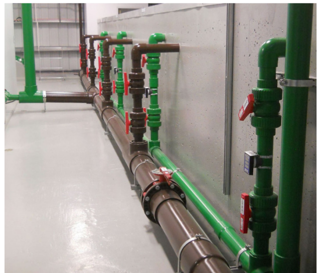
Showing the inlets to filters (green pipes) and the outlet of wastewater from the filters (brown pipes)
