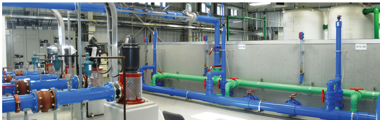
View of treated water outlet from the filters (blue pipes) and water for filter maintenance (green pipes). Distribution pumping in the foreground.
