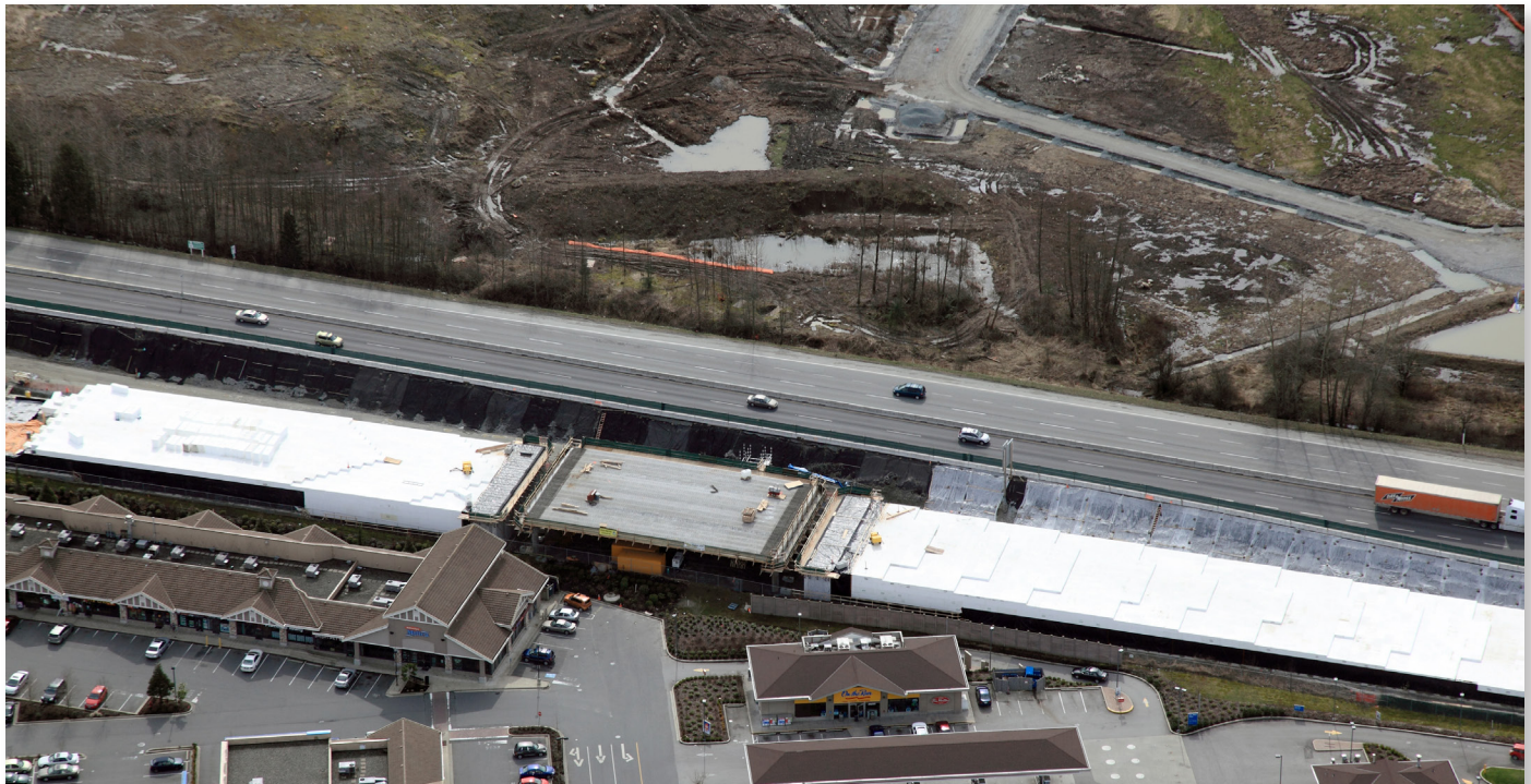
March 20, 2011 - 202 St at Highway 1 looking south toward Trans Canada Highway. Eastbound traffic detour in place; Westbound lanes under construction including EPS approach fills and westbound overpass structure. Original wetland visible on south side of TCH.
