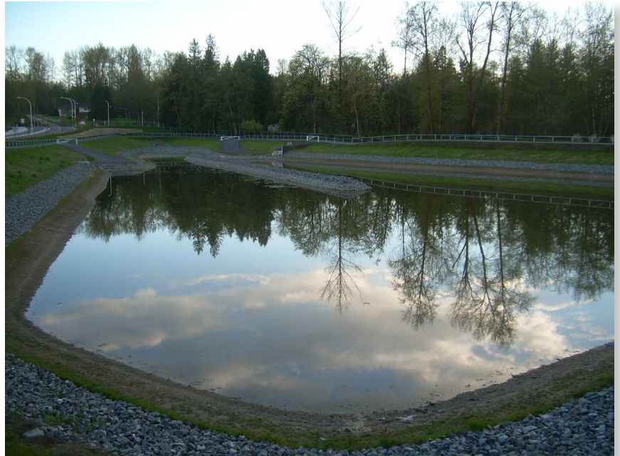
April 2013 - Retention Pond looking south; 202 St in left background. The pond was constructed to be hydrologically functional one year prior to project completion.
