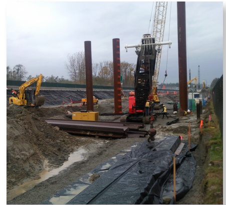
October 28, 2010 - Westbound piles splicing, looking west from atop north side pre-cast EPS perimeter foundation.
