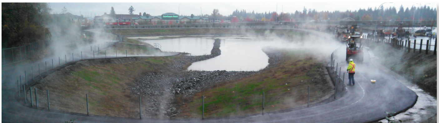
Installation of hot asphalt upon the multi-use path atop the retention pond.
