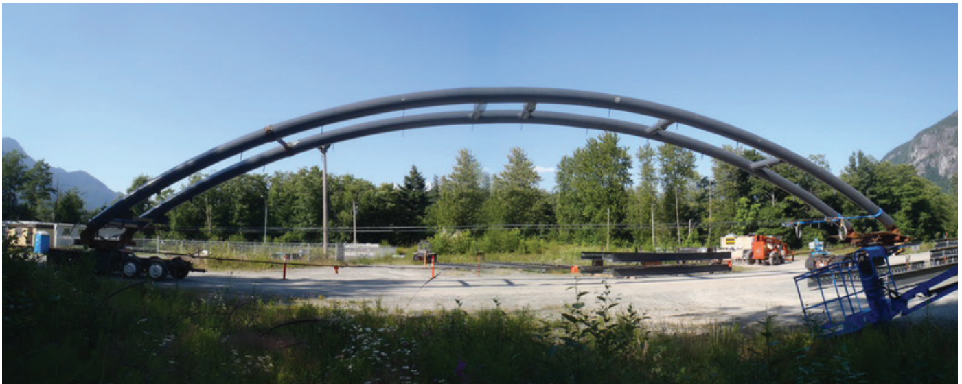
The fully-constructed steel arch awaiting installation on site. The blue-grey colour of the arch represents the story of the “great flood” in Squamish folklore.
