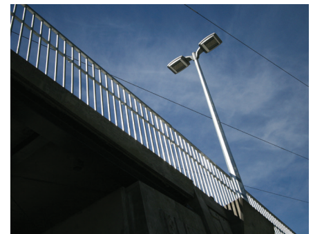
LED lighting is installed along the bridge approaches in addition to down lighting on the thrust walls.
