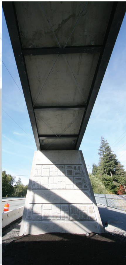
The jump span and east approach ramp allow for long-term settlement and full view of the pier's artwork.
