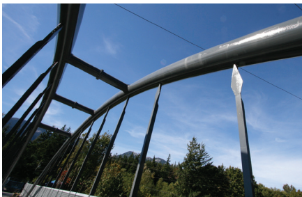
The spear heads for the hangers mask the bolted connections from view. The carefully chosen count of 16 spear-heads represents the 16 hereditary chiefs of the Squamish Nation.
