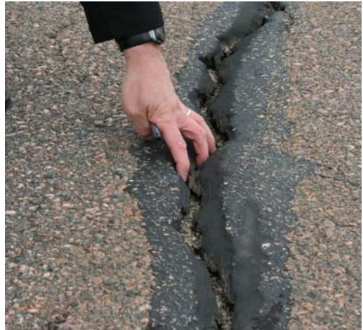
*Transverse Cracking had occurred on the existing runway in several locations. It appeared that the runway had deteriorated over time due to thermal loading.*
