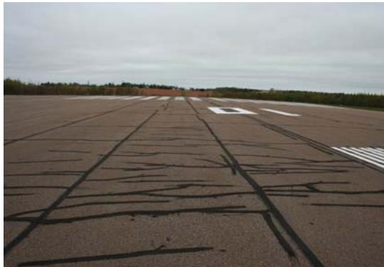
*Longitudinal, transverse and joint cracking were prevalent on the pre-existing runway*
