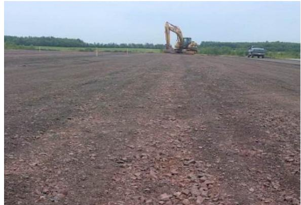
*The base aggregate following the milling of the existing asphalt surface. Innovation to handle the poor gradation and surficial aggregation saved not only budget and schedule but the carbon emissions that would be caused from additional hauling and equipment operations.*
