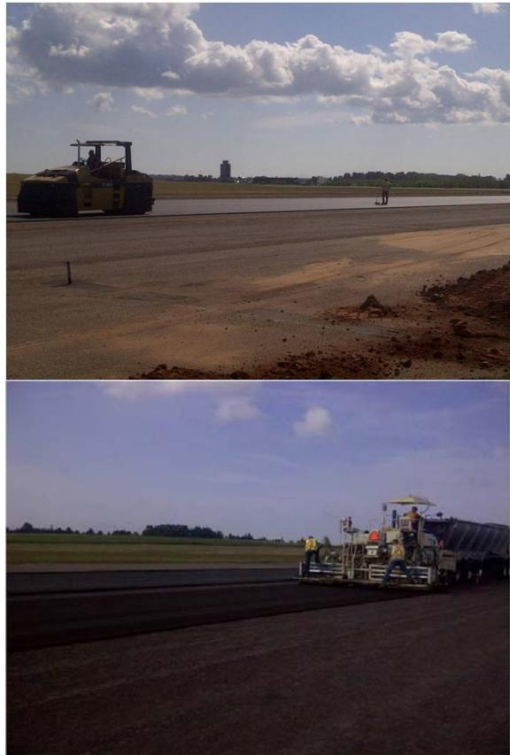
*The recycled asphalt millings were spread onto the pre-compacted rough aggregate base. The millings were then compacted onto the aggregate base following application*
