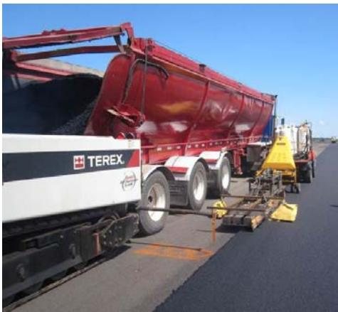
*Paving was completed using asphalt joint heater. The paving schedule was in jeopardy when rain occurred during confined window for construction. A portable heater borrowed from a nearby ice arena helped to dry materials so paving could proceed as planned.*
