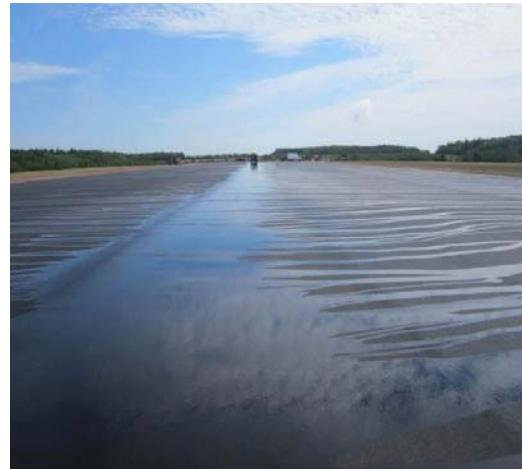
*At the end of the project, flood tests were conducted to identify any ponding areas. The project went very smoothly and was completed on budget and on schedule.*
