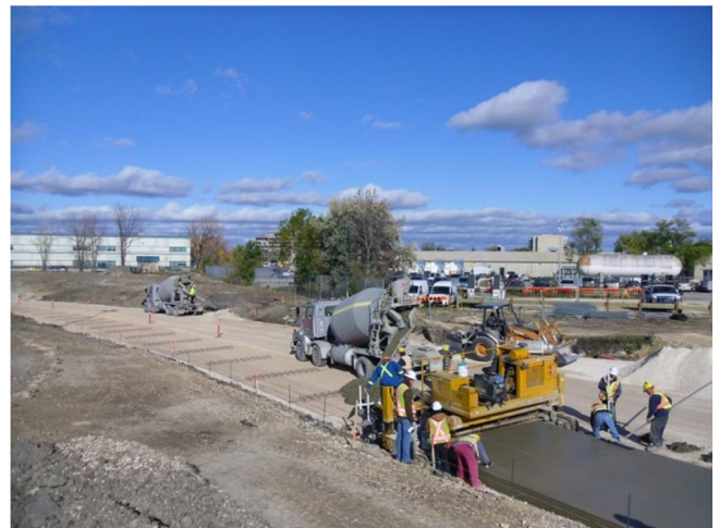
Figure 9 – Slipform Paving of Transitway
