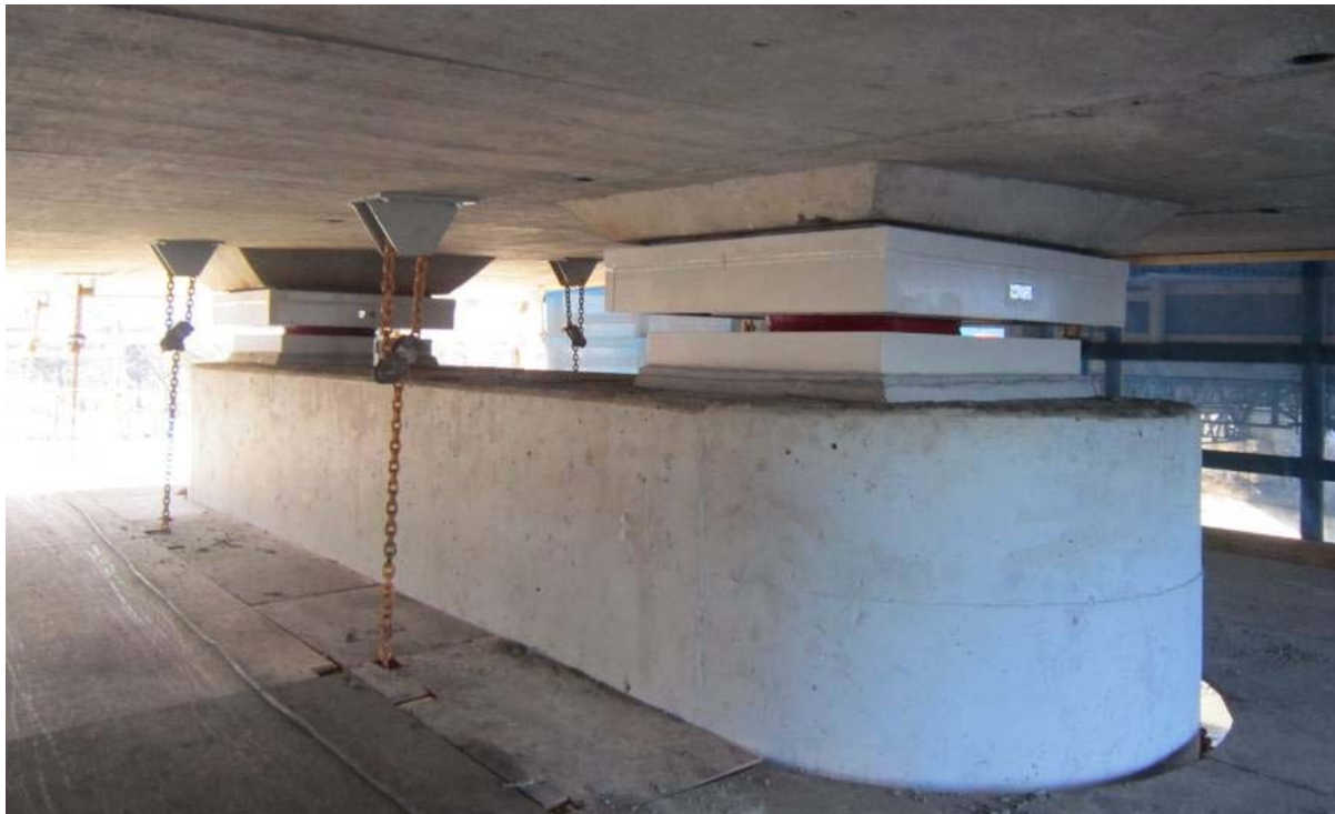
New seismic isolation bearings
