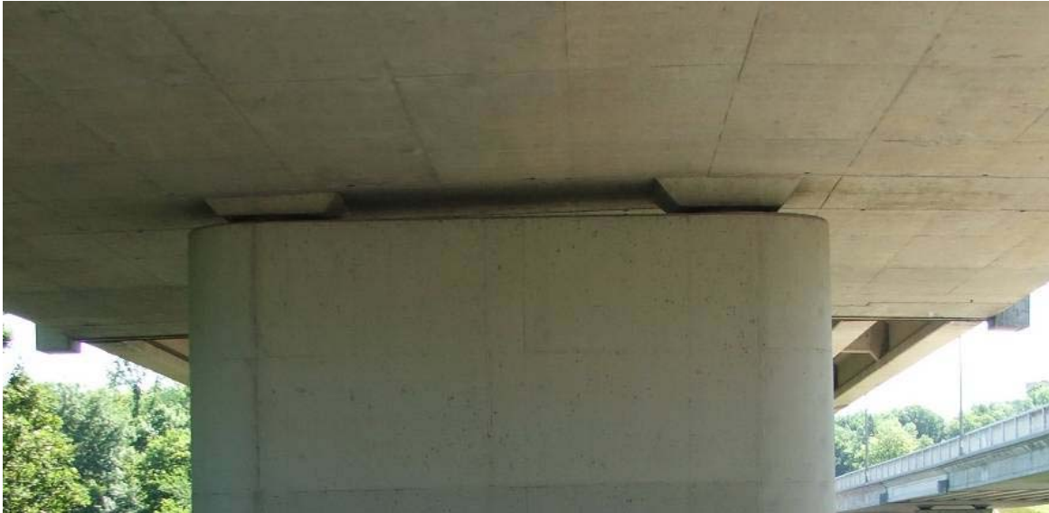
Existing bridge bearings
