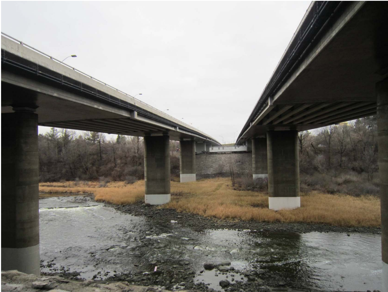
Overview of retrofitted bridge with new seismic isolation bearings and new external post-tensioning system
