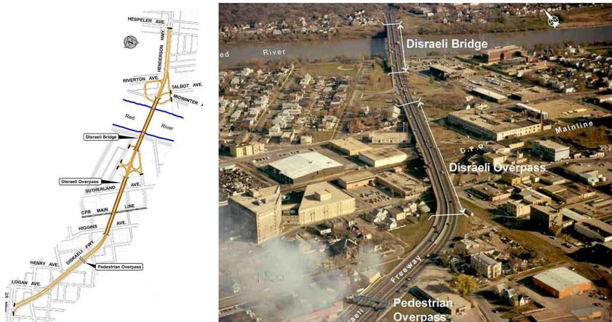
Figure 1 – Existing Disraeli Facility
