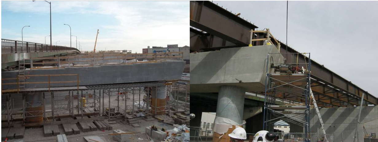
Figure 6 – Post-Tensioned Pier Cap
