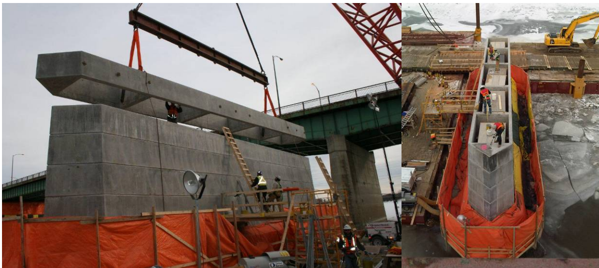
Figure 5 - Construction of River Piers
