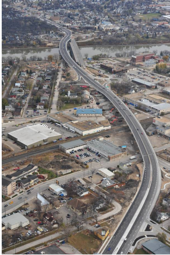
Figure 7 – Completed Disraeli River Bridge and CPR Overpass
