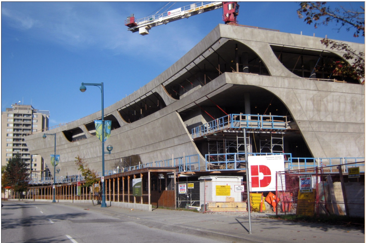
Figure 7: Construction of self-supporting cast-in-place concrete exterior cladding walls. Photo Credit: Stephan Pasche
