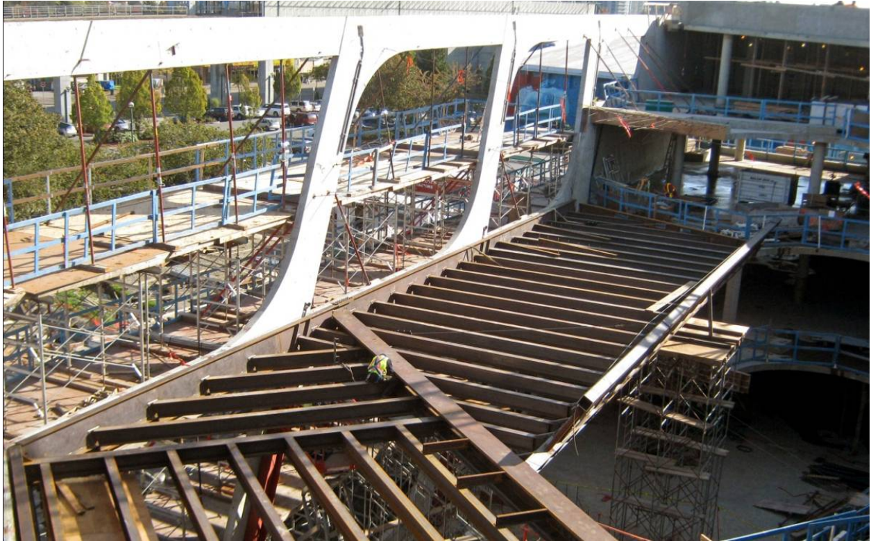
Figure 4: Construction crews assemble third floor steel, inside the cast-in-place cladding. Photo Credit: Fast + Epp
