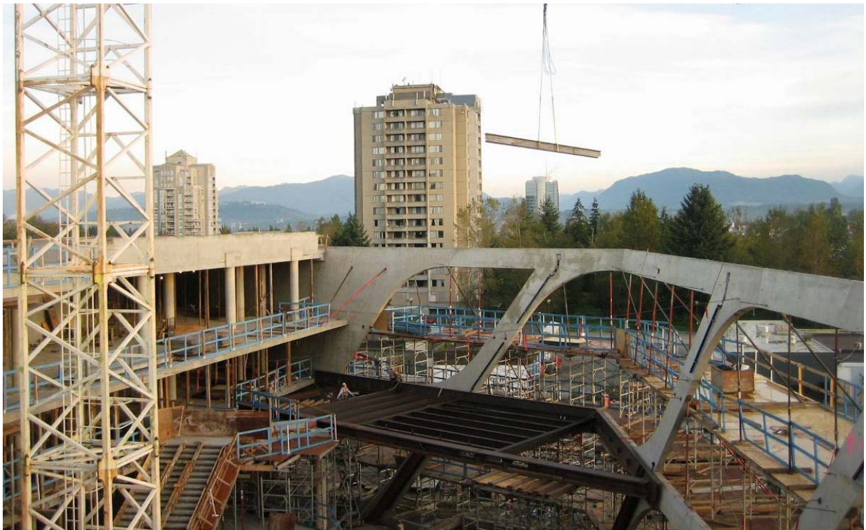
Figure 3: Construction crews assemble third floor steel, inside the cast-in-place cladding. Photo Credits: Solid Rock Steel
