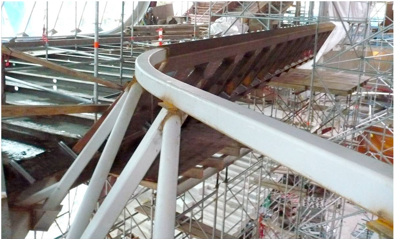
Figure 10: Rounded corner of the tilted truss follows geometrical form of Surrey City Centre Library's interior guardrail and supports much of the building's third floor. Photo Credit: Fast + Epp
