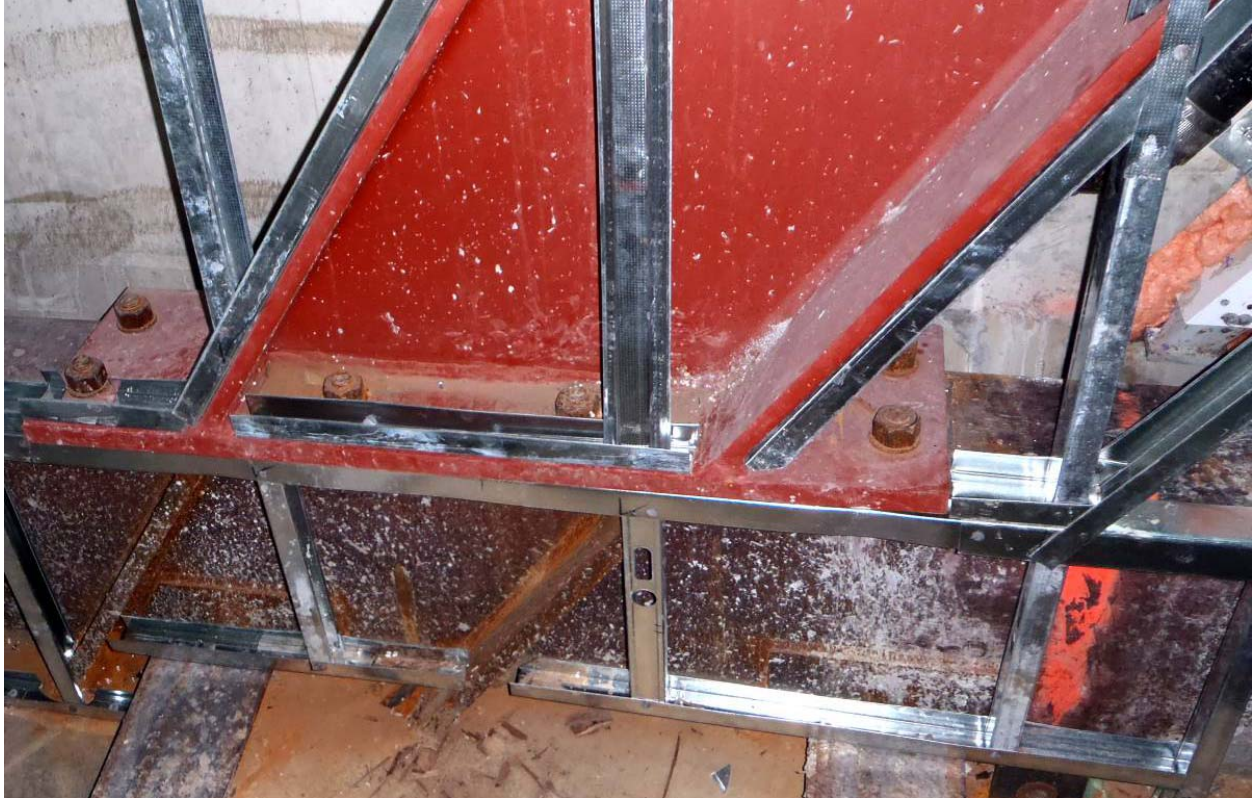
Figure 9: Close up of tilted steel column that supports third floor and roof atrium structure, which will be concealed behind drywall. Photo Credit: Fast + Epp
