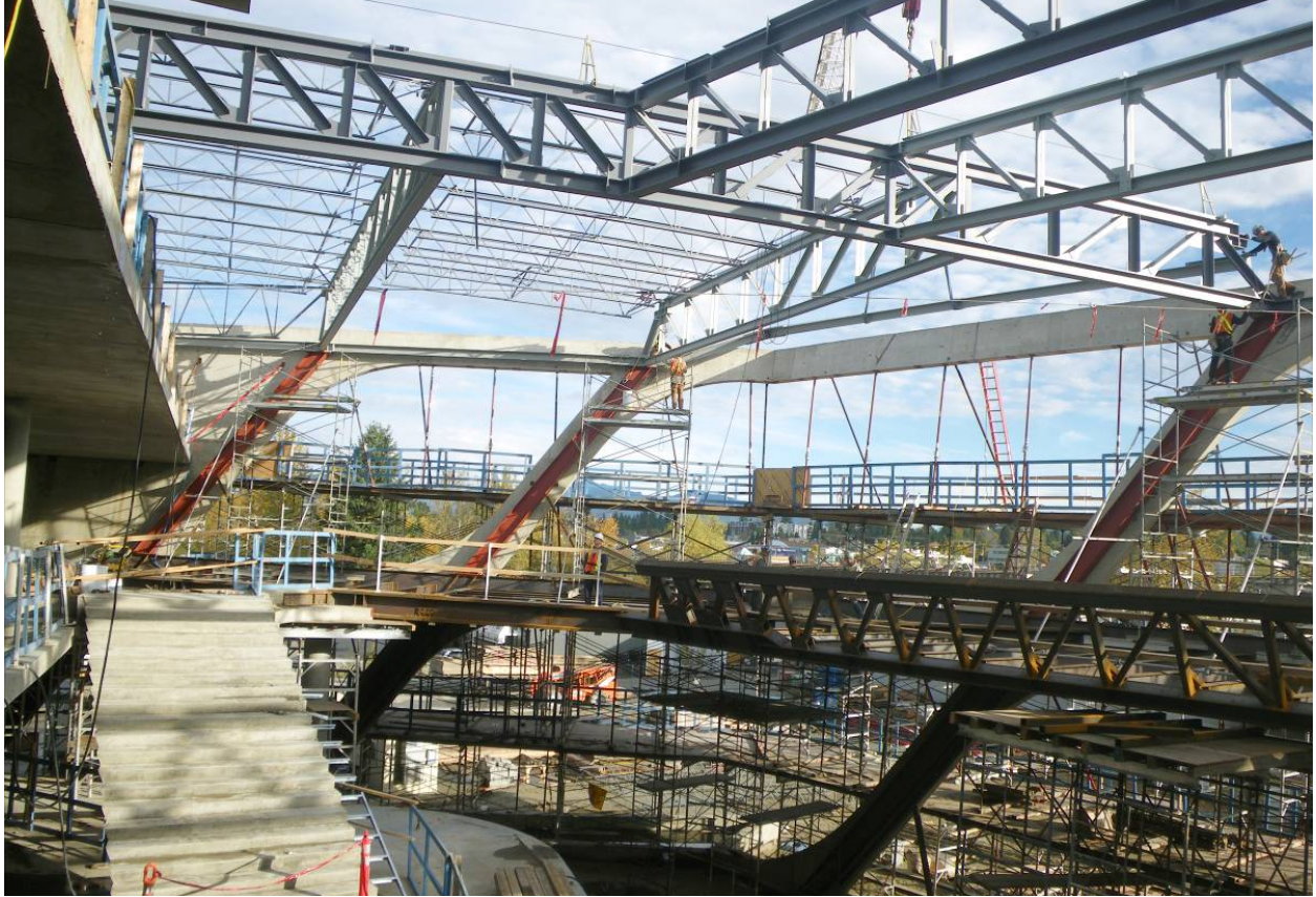
Figure 11: Steel roof trusses allowed the atrium to remain column free and support the tilted skylight pop-up. Photo Credit: Fast + Epp
