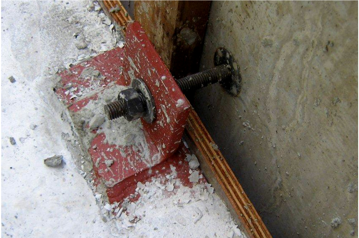
Figure 6: Custom seismic connectors, developed to carry the significant gravitational and seismic loads. Photo Credit: Stuart Olson Dominion Construction Ltd.
