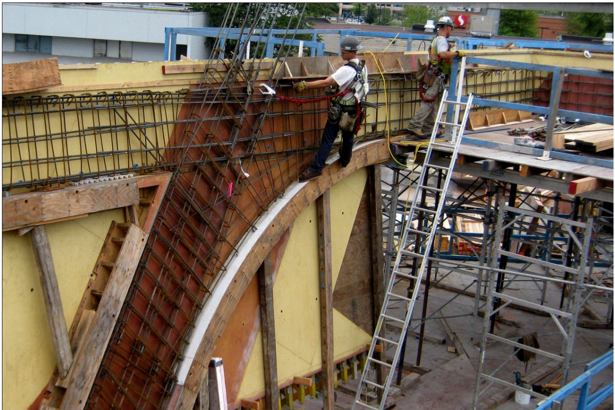
Figure 5: Complex geometry required careful rebar detailing. Photo Credit: Lawrence Chan
