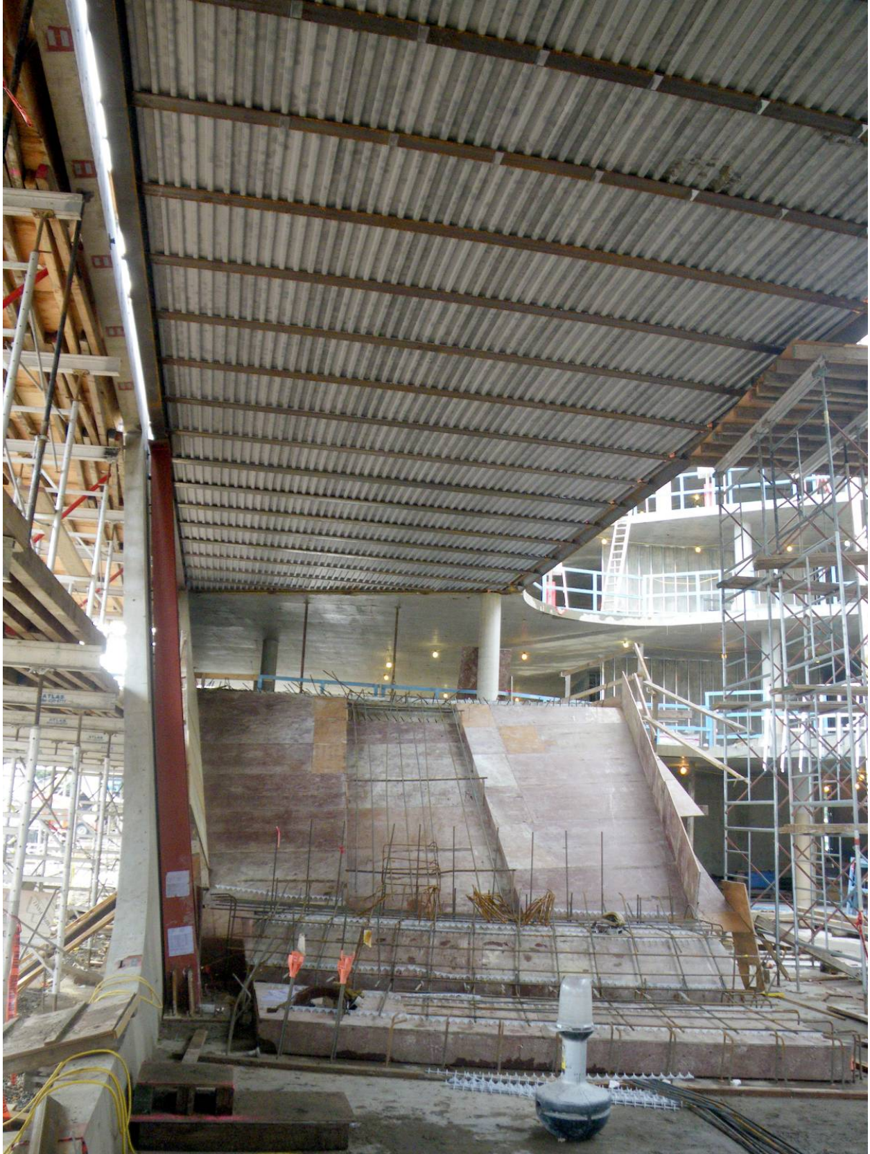
Figure 8: Underside of steel decking showing flush steel beams to reduce the floor depth. Also shows tilted steel column in tight tolerance to concrete cladding. Photo Credit: Fast + Epp
