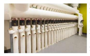
Significant effort was made to carefully calculate the system equilibrium in order to ensure that it operates optimally under all possible operating conditions including peak summer and winter conditions as well as mid-season conditions. As such, the system is solicited at its maximum throughout the year. Also each geothermal well is independent from all the others in order to minimize any negative impacts on the capacity of the system in the event of a failure of one of the wells.
