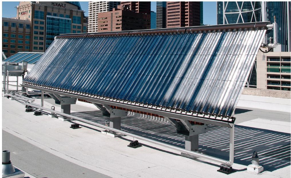
Rooftop solar hot water system
