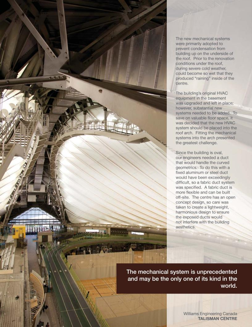
Various types of fabric duct were researched and a Danish supplier was identified to supply a patented system of fabric ducts and jet-throw nozzles. The nozzles are attached at specified intervals, on the eleven o'clock and the two o'clock positions of the fabric duct, and direct air to the underside of the roof in a complex and specific pattern.
