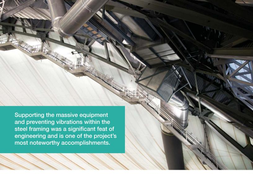
Two, 45,000 CFM fans were installed in the arch and required additional structural support for positioning into the architectural elements of the building. Supporting the massive equipment and preventing vibrations within the steel framing was a significant feat of engineering and is one of the project's most noteworthy accomplishments.
