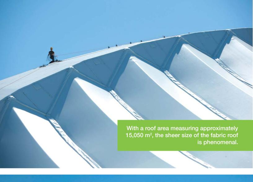
The first thing anyone notices about the Talisman Centre is its striking white fabric roof. A sculpted, tent-like form, the roof descends in a series of panel ridges from a large arched spine. It measures approximately 15,050 square metres in area. The roof is a unique aspect of the building both aesthetically and in function.
