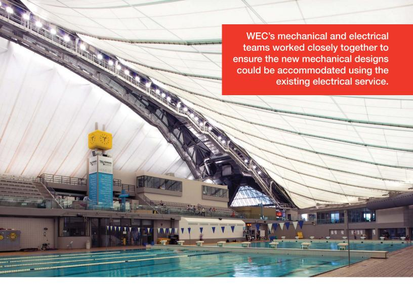
Existing pendant lights over the pool presented both maintenance and accessibility difficulties. Each time a lamp or ballast required replacement, the pool had to be emptied. Therefore, these fixtures were removed and replaced with indirect metal halide and fluorescent lights which were added around the ring beam on the structural supports for the fabric duct.
