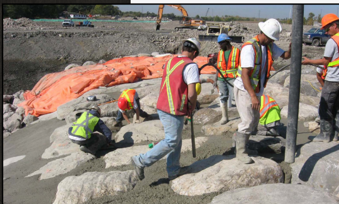
Placing boulder concrete (September, 2009)
