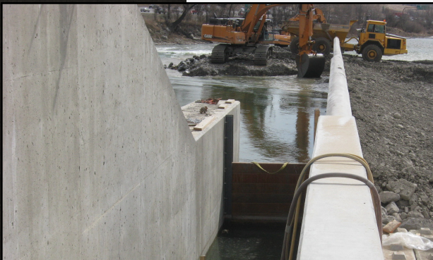
Extension of fishway wall (April, 2009)
