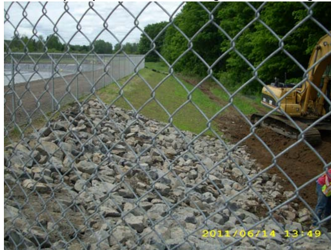
Figure 12: Rip Rap for Protection Against Flooding Events
