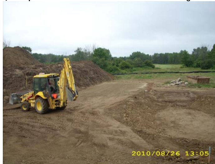
Figure 6: Fueling Pad (center), Silt Fences (background) and Sedimentation Pond (right) - Implementation of Environmental Management Plan
