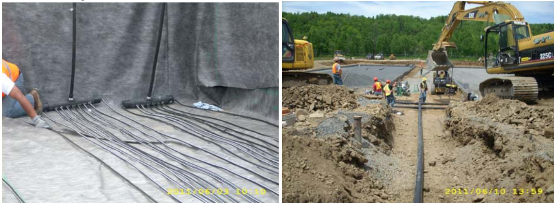
Figure 9: Installation of Air Headers for Both Chambers of SAGR
