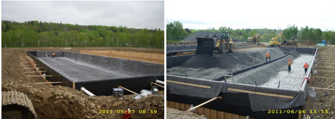
Figure 7: Construction of SAGR Chamber
