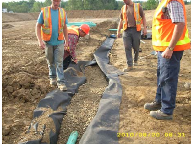
Figure 3: Sub-Drainage System - Aerated Cell
