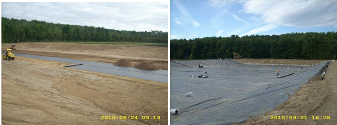
Figure 4: Geotextile and Sand Base Preparation for HDPE Liner - Aerated Cell
