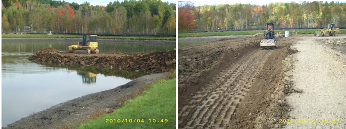
Figure 5: Construction of the Dividing Dike - Imported Clay Material
