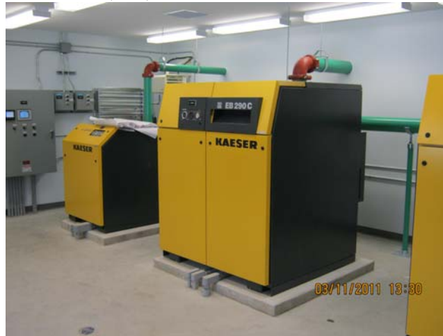
Figure 10: SAGR Blower (left) and One of the Aerated Cell Blower (center)
