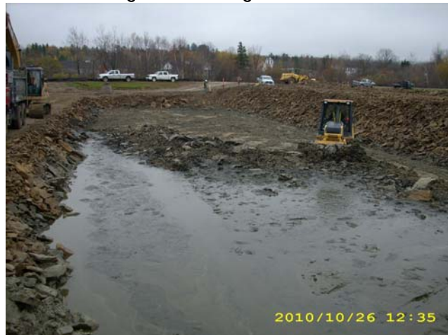
Figure 2: Sludge Removal
