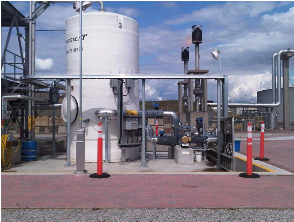
Photo 3: Heat Traced and Insulated Feedstock Storage Tank; the digester gas flare is in the background.
