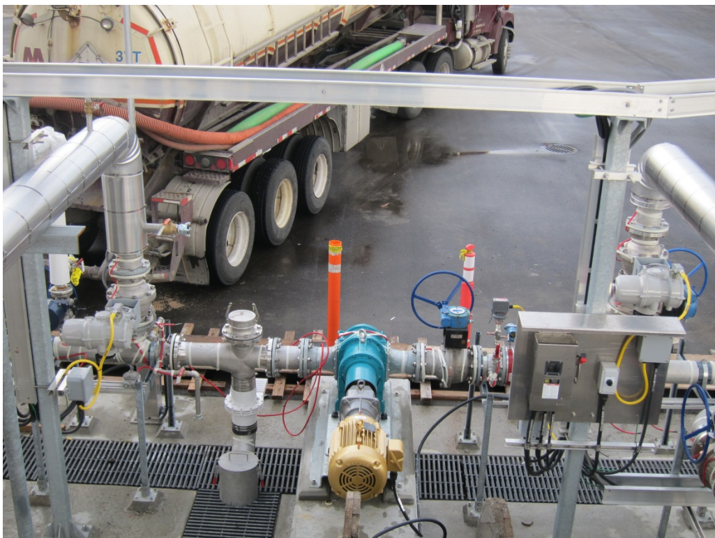
Photo 7: Feedstock Unloading Pump and Piping Undergoing Testing
