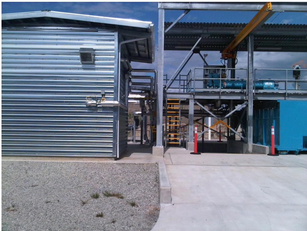
Photo 4: Co-digestion Operations Building / Utility Shed; the Parkson Sludge Strainer for thickened primary sludge and screenings bin are illustrated also.
