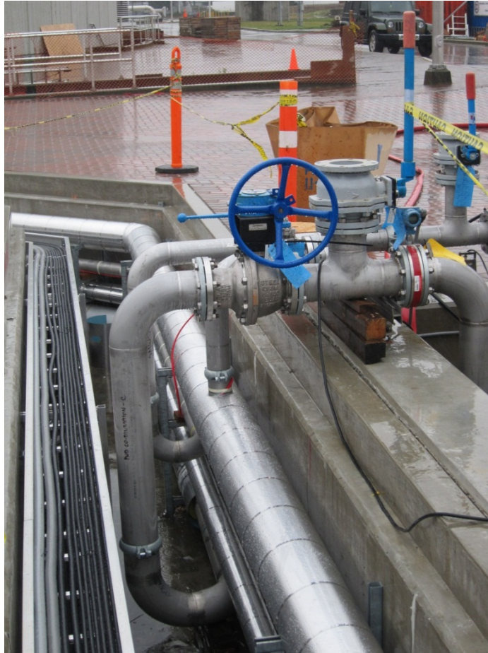
Photo 5: Utility Chase to Convey Piping and Cables to/from Digesters
