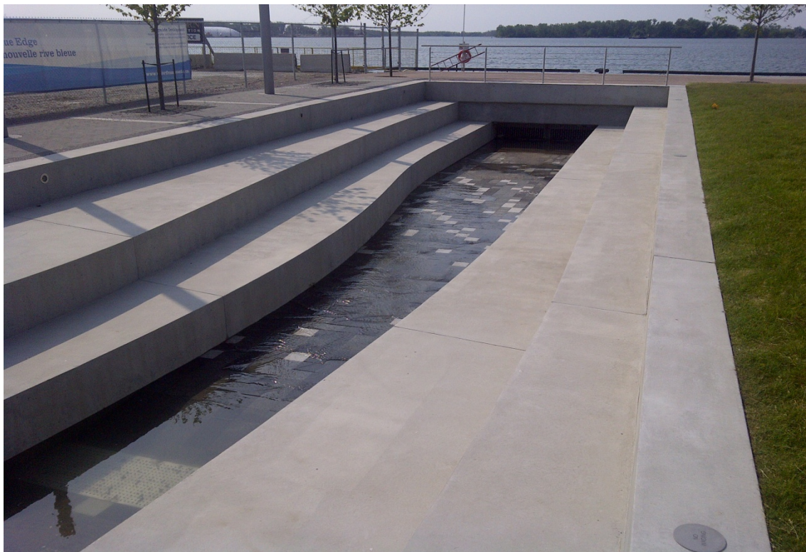
8. Outlet to Lake Ontario, Re-circulation Intake Grate in Foreground
