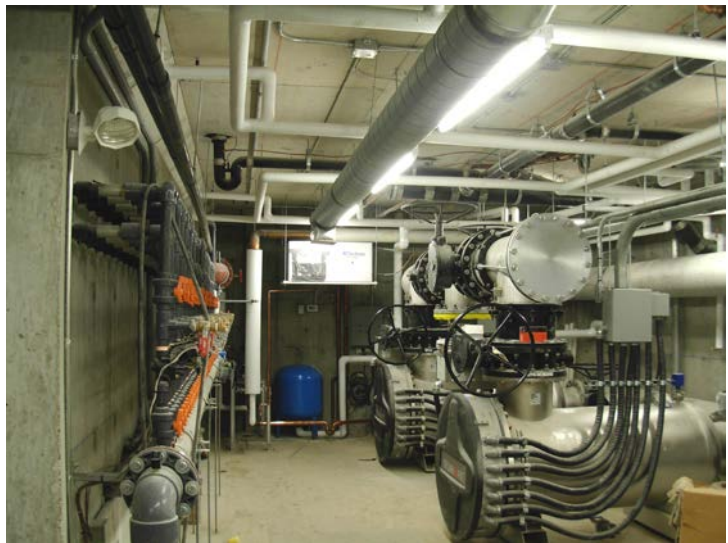
UV Treatment Units used at Sherbourne Common
