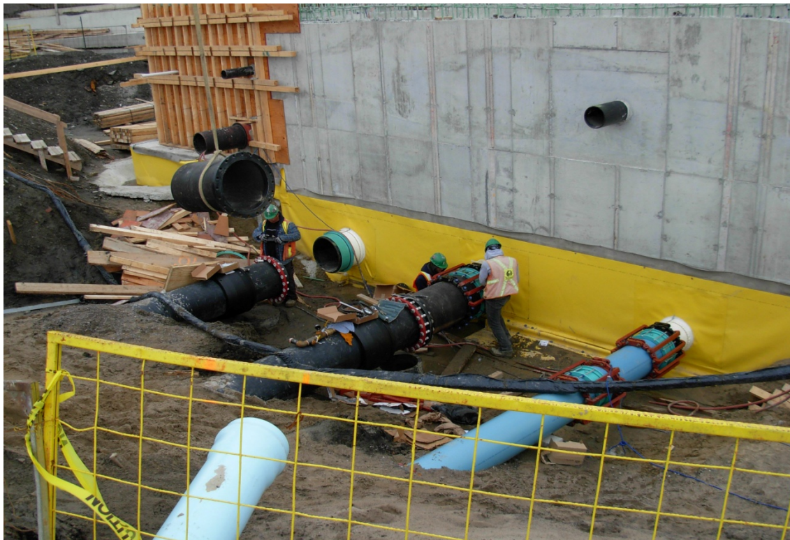
2. Construction of Intake Pipes into Wet Well
