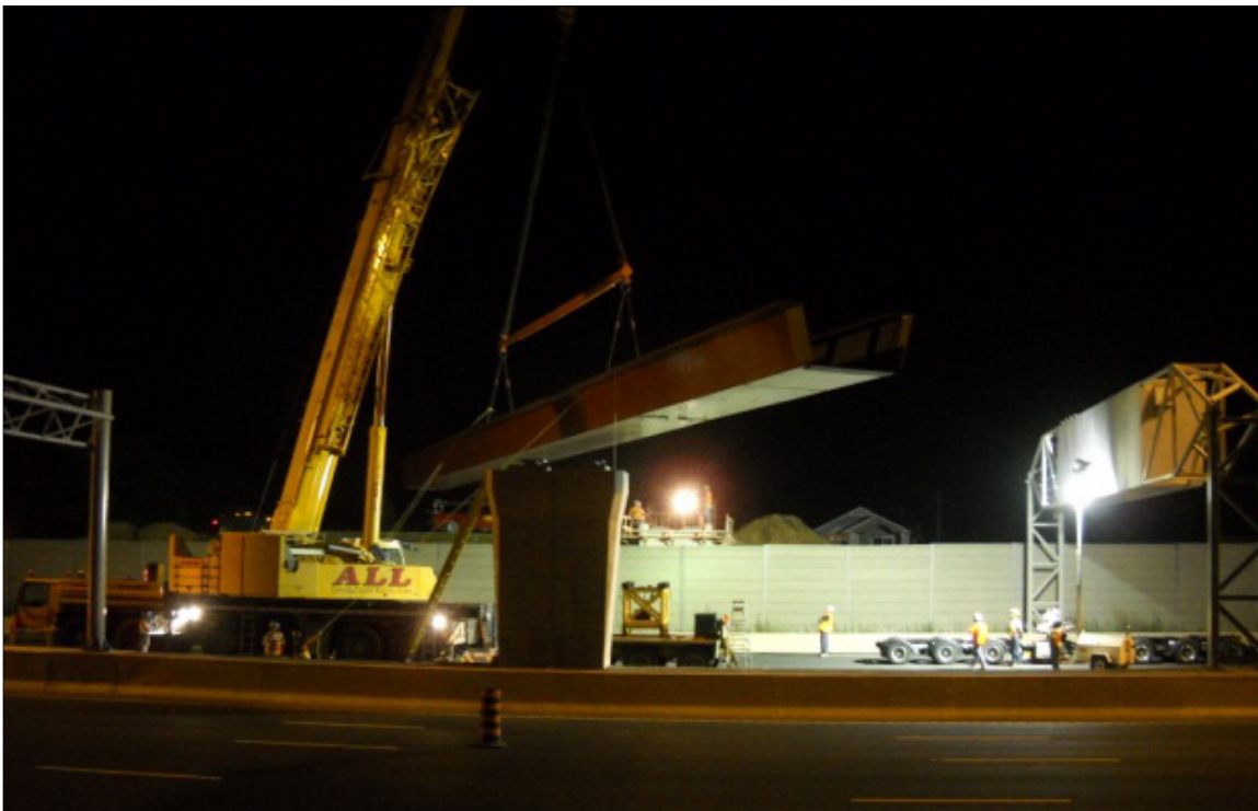
Erection during Night-Time QEW Closure Photo Credit: McCormick Rankin Corporation
