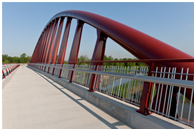
Figure 7: View of Inclined Arch Rib
