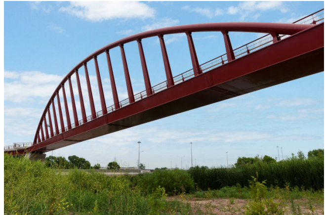
Figure 6: View of Tied Steel Arch Span
