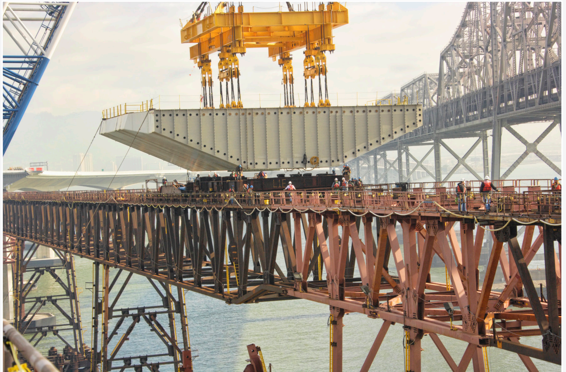
Staged analysis was required to verify structural integrity and geometry to tolerances within millimeters
