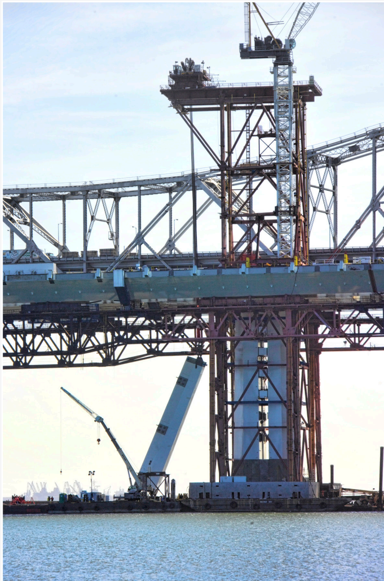
Single steel tower required an independent temporary tower to lift the components into place
