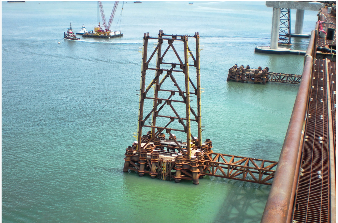
Completed tubular EBF tower on deep marine foundation driving frame
