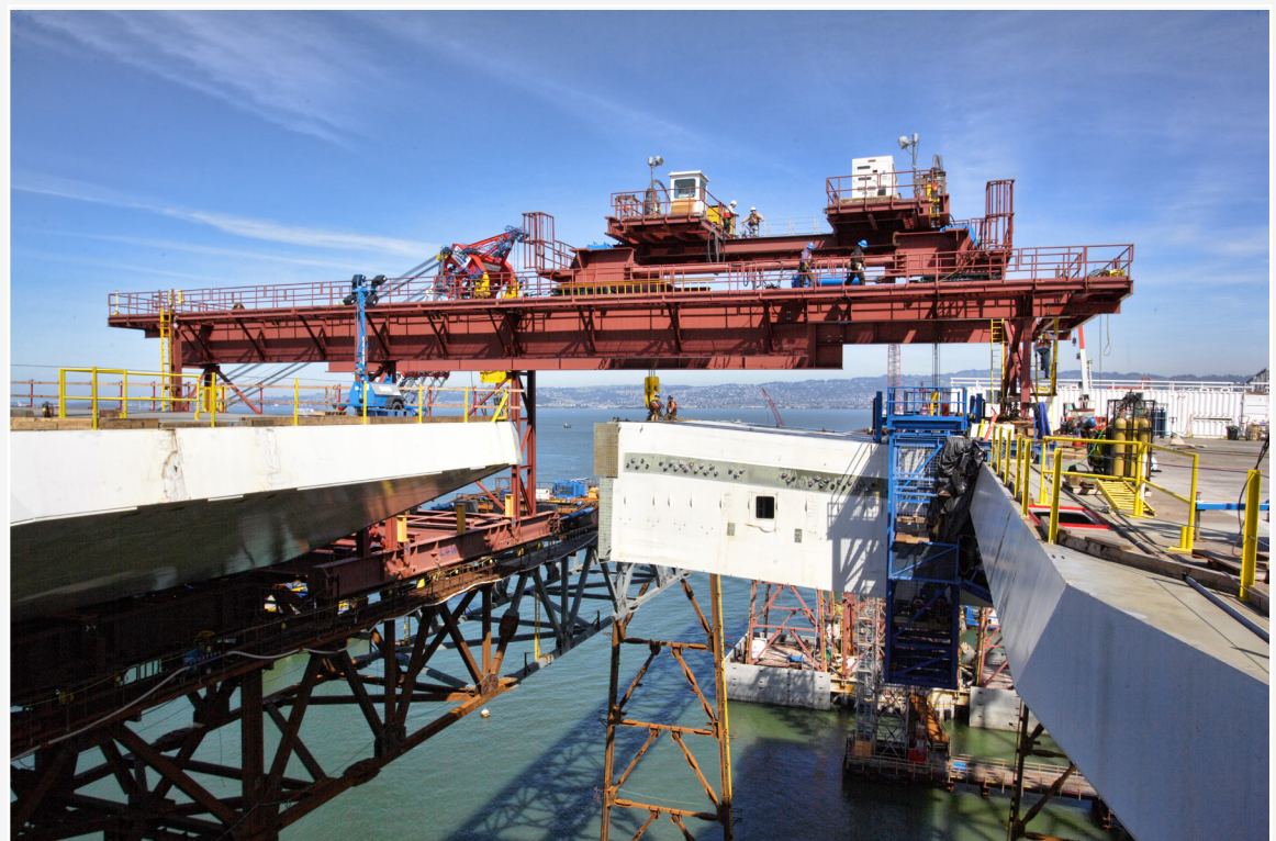
Crossbeam connection - one of 47 individual segments lifted and connected
