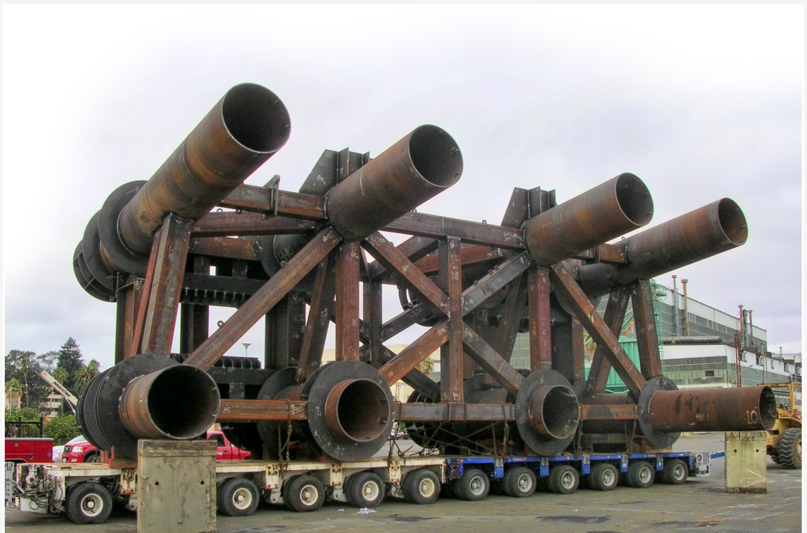
Overland transport of marine foundation frame
