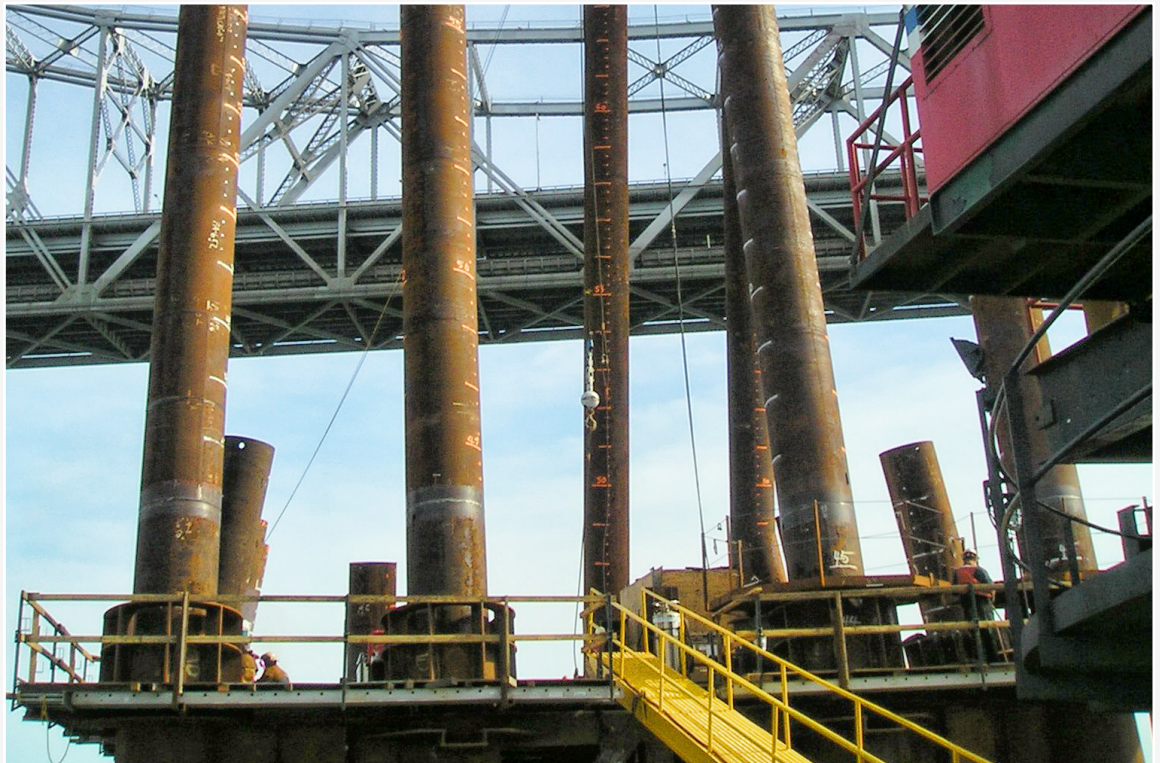
Piled tower foundations in “bay mud” in 25m deep water
