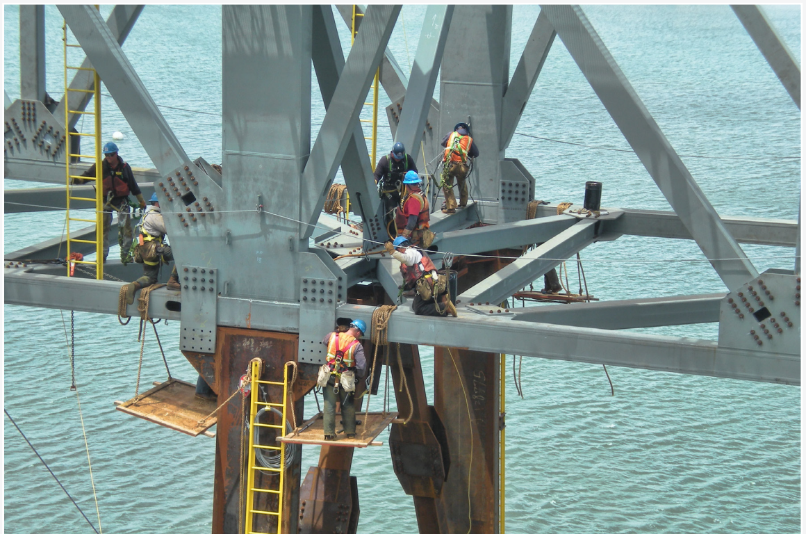
8.5m deep temporary trusses lifted and placed with marine crane
