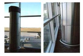
The third critical area is the passenger holdrooms. These areas incorporate both a continuous band of jet diffusers and a series of stainless steel 'totems'.
