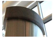
A series of "eyeball" diffusers located below the clerestory windows in the departures hall jet small volumes of air at a high velocity causing air movement with minimal use of fans.
