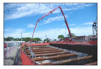
Installation and Removal of the Shoring System – Due to the depth of excavation required, close proximity of the CN rail tracks and the narrow constraints on site, a shoring system was required to be designed and implemented prior to the installation of the tunnel structure. The Contractor, together with Dillon, devised a shoring system that included sheet piling located on three sides of the tunnel structure and struts that spanned between the sheet piles. Sheet piling
