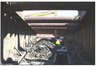
place to support the shoring. It was critical that the Contractor was to maintain conditions and protection of the CN railway tracks and ensure that work activities did not at any time jeopardize the stability or impact the performance of the tracks.
