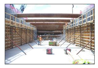
**Walls** – The walls range from 900 mm to 1000 mm in thickness. Because of the fixity with the bottom slab, most of the reinforcement is required at the bottom of the outside face in order to carry moments transferred around the corner from the bottom slab. The walls were designed with temporary openings to allow the open excavation to be braced across during construction. After the bracing is removed, these openings will be sealed.
