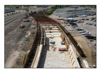
Due to the property constraints mentioned earlier, the tunnel intersects the tracks at a very large skew angle. This skew made avoiding interference with the tracks during construction much more difficult than if the crossing was aligned perpendicular to the tracks. A detailed description of the tunnel design follows.
