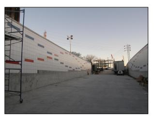
**Interface Wall** – One of the main concerns during the pre-design was the transition of the construction sequencing between Stage 1 and Stage 2 structures. This area is called the interface wall. As a result, several solutions were incorporated into Stage 1 of the design.
