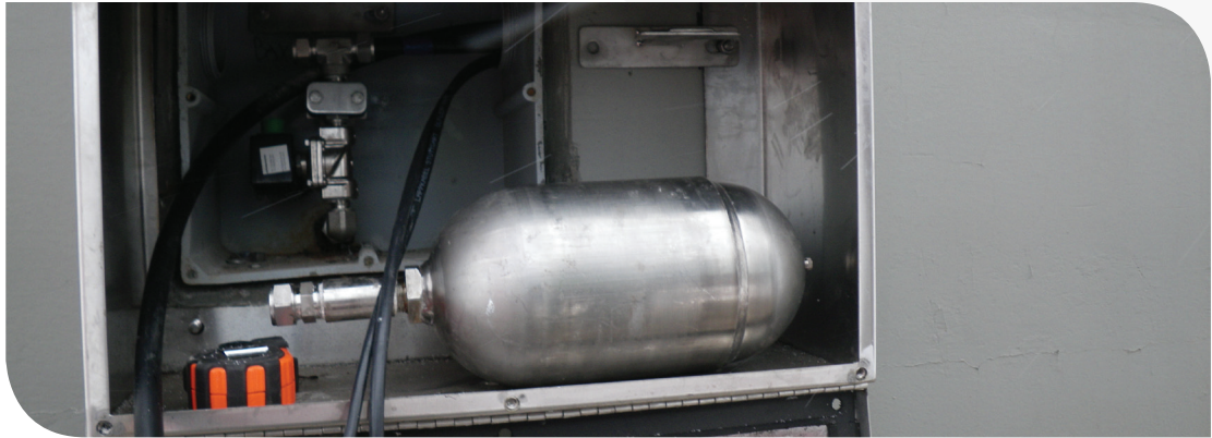
Road side pressure tank and valve
