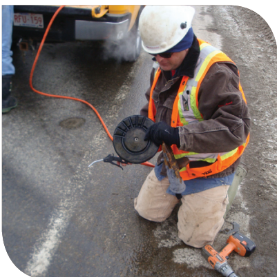
Final spray disk adjustments
