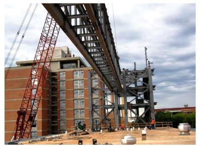
process. The contractor summed up the situation best, "We built a protective platform over the existing structure to protect the roof and its occupants, and we covered the walkways into the building to keep people safe. The construction area went beyond the existing structure's footprint and above. We started with the east and west towers and built up to the eighth floors, and then we began erecting the trusses for each floor.
