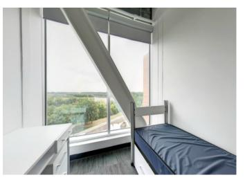
construction. While highly unusual, exposing the robust exterior truss members within the modestly-sized residence rooms created a dramatic design, which accentuated the need to incorporate artful structural design details.
