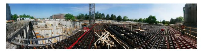
When we began the project, our schematic design identified reinforced concrete as the best option in terms of its ability to provide a robust and economical structure. Concrete was also adopted for aesthetic reasons, with the architect choosing to express architectural concrete columns and slab soffits around the day-lit perimeter of the building.
