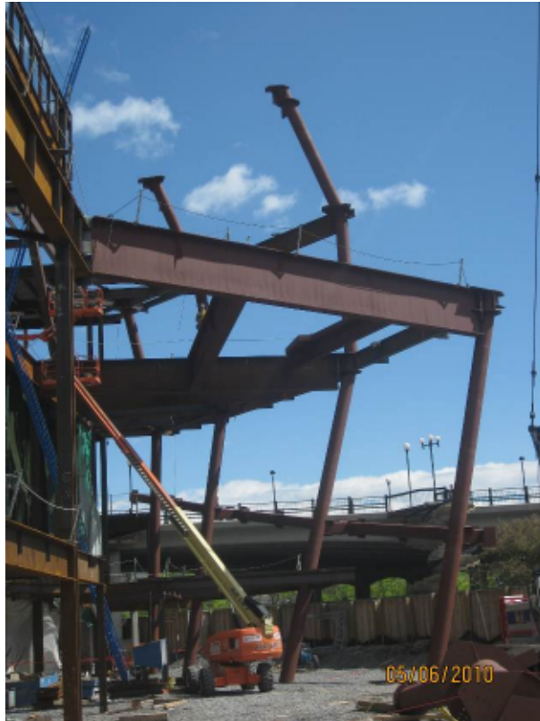
Figure 10: Level 3 Pre-Function Sloped Columns
