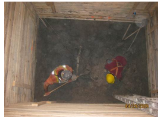
Figure 9: Hand Excavation in Existing Parking Garage
