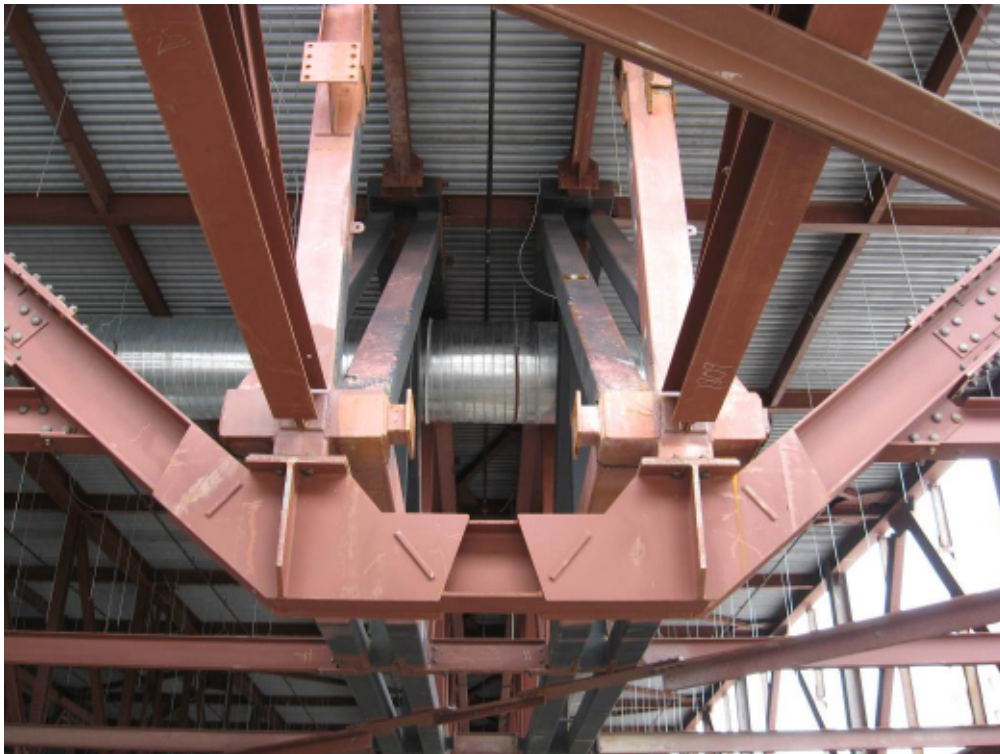
Figure 11: Roof Cradle Truss Supporting Existing
