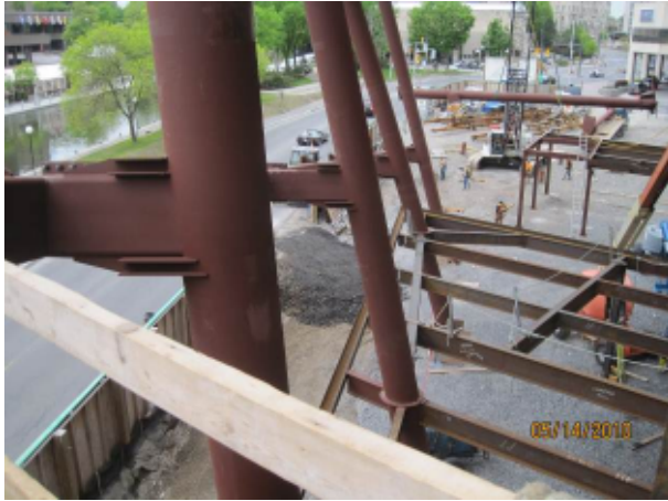
Figure 15: Sloped Columns @ Keel Beam Level
