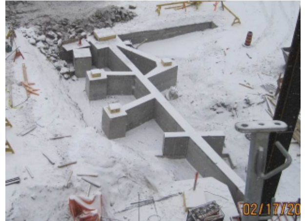
Figure 16: Sloped Column Compression Strut
