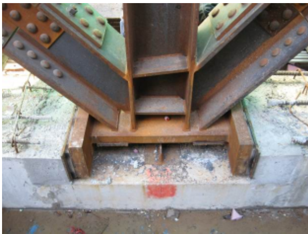
Figure 14: BF4 Vertical Slip Joint at Horizontal Concrete Drag Beam
