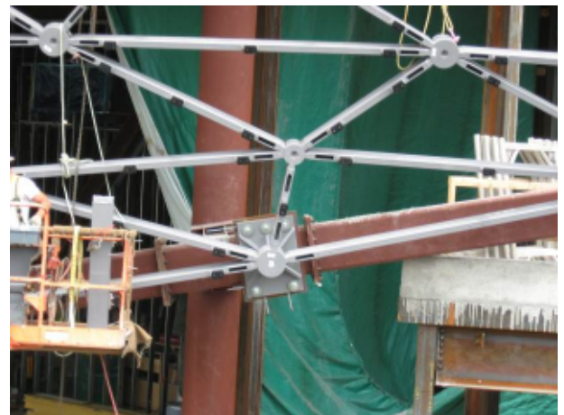
Figure 18: Glass Wall Connection to Keel Beam
