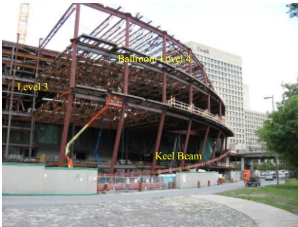
Figure 17: Front Façade Support Structure
