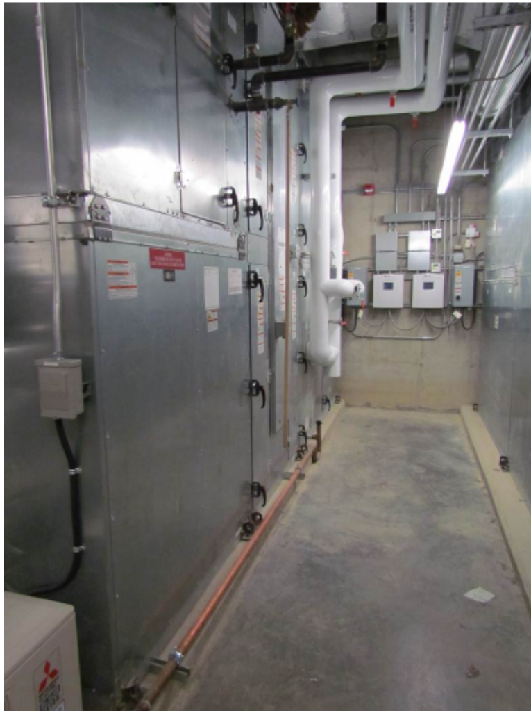
Air Handling Unit and Variable Frequency Drives for Fans and Pumps
