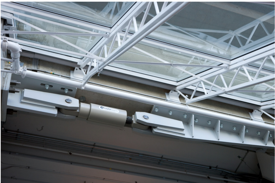
Circumferential Viscous Damping Device at Expansion Joint – Level 4
