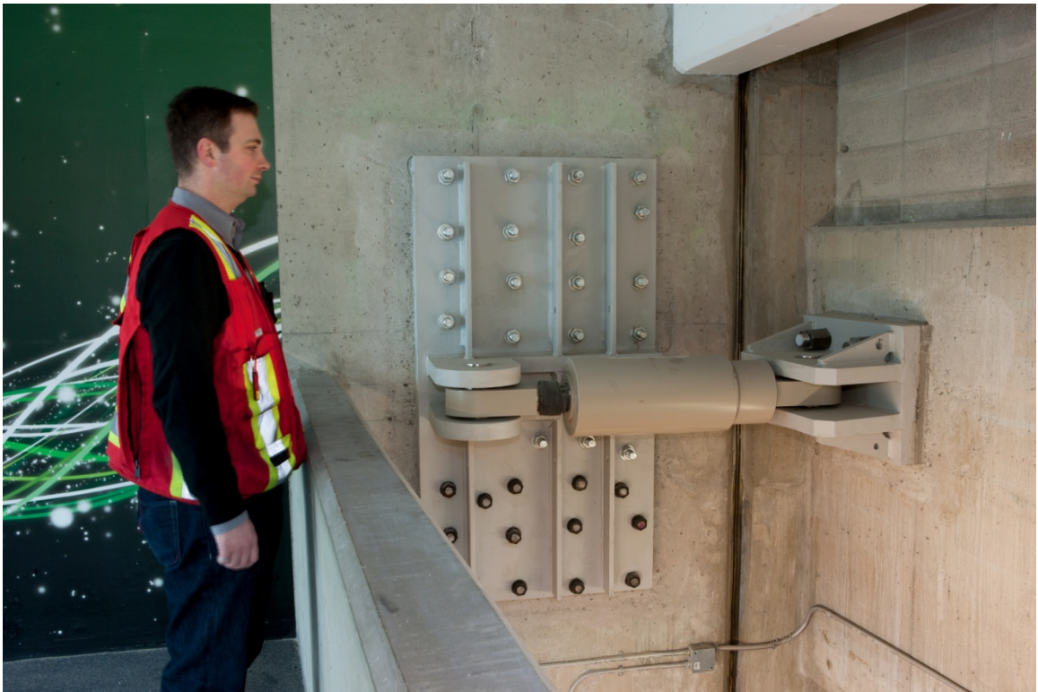
Radial Viscous Damping Device at Ramp Wall
