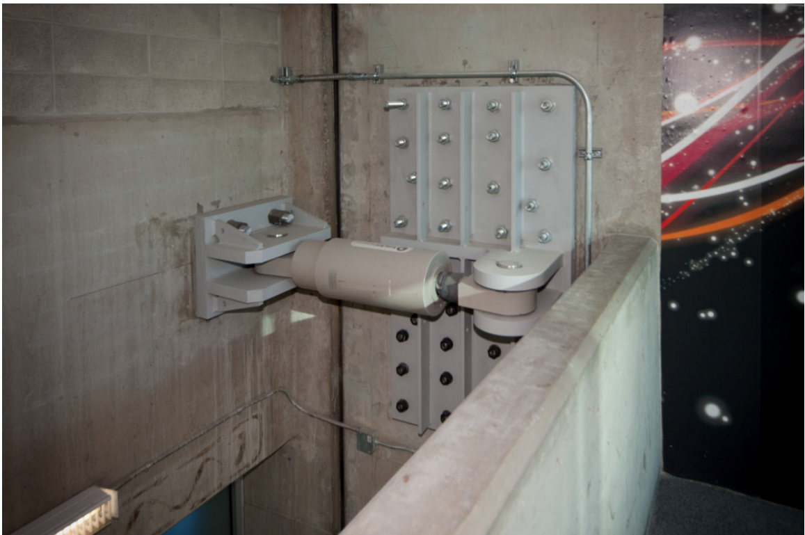
Radial Viscous Damping Device at Ramp Wall
