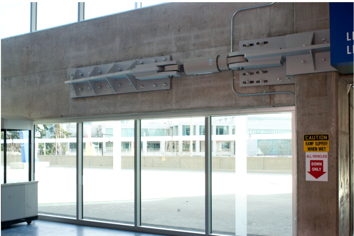
Circumferential Viscous Damping Device at Expansion Joint – Level 2
