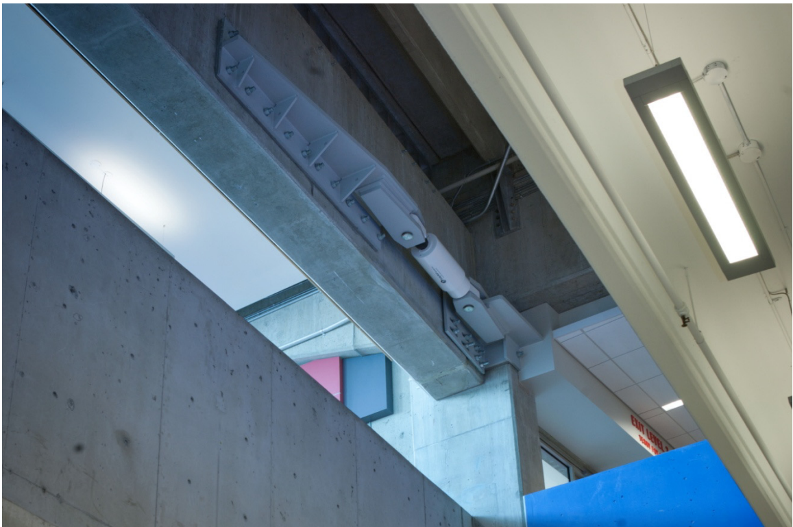
Circumferential Viscous Damping Device at Expansion Joint – Level 3
