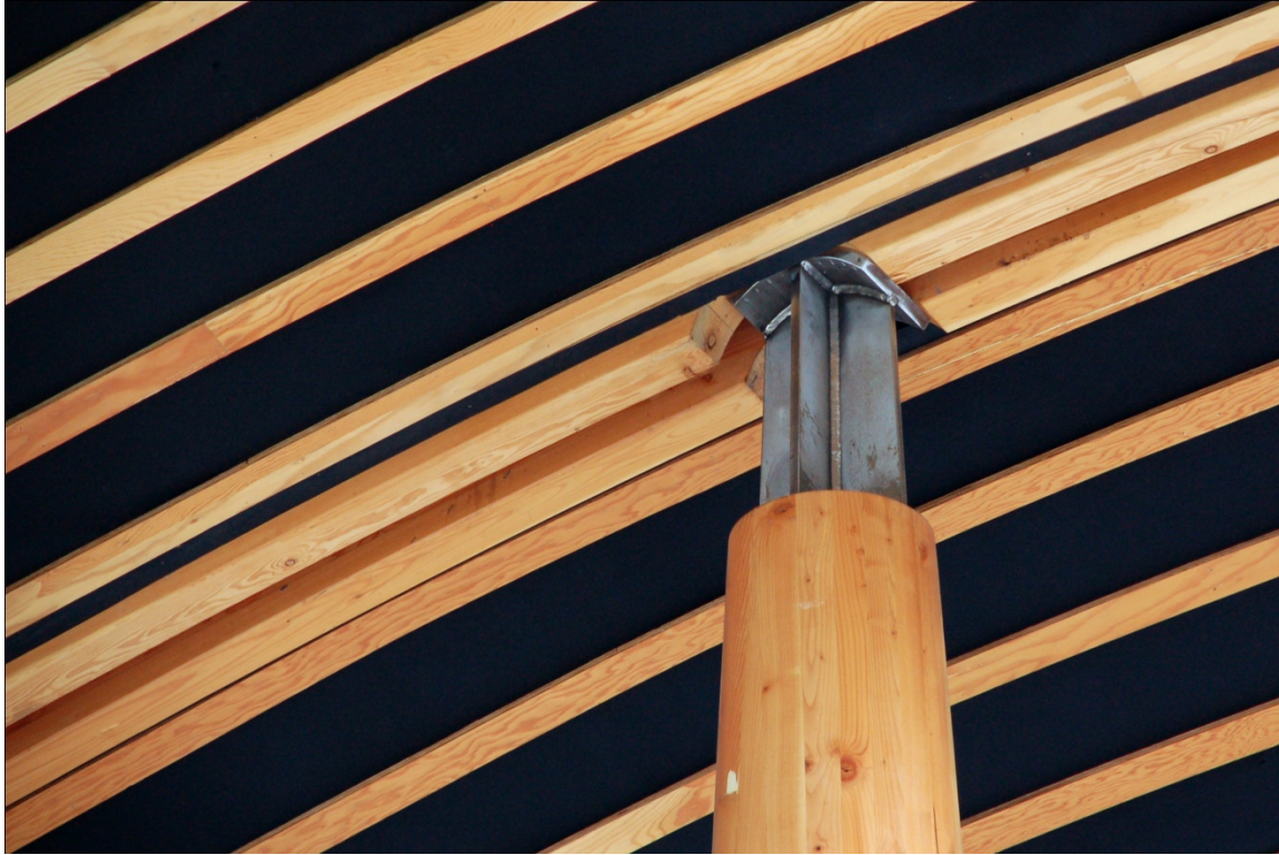
Figure 5 – Novel universal panel-to-column connections.
