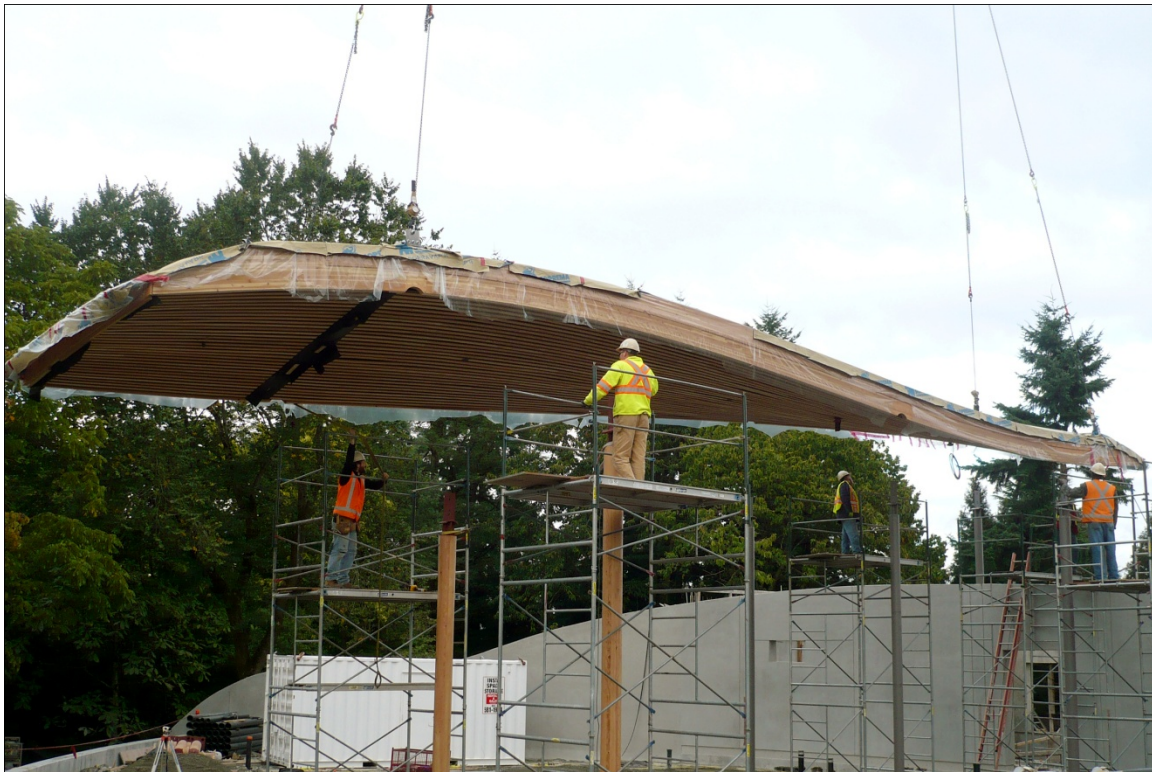
Figure 8 – Crews begin assembling prefabricated panels on site.
