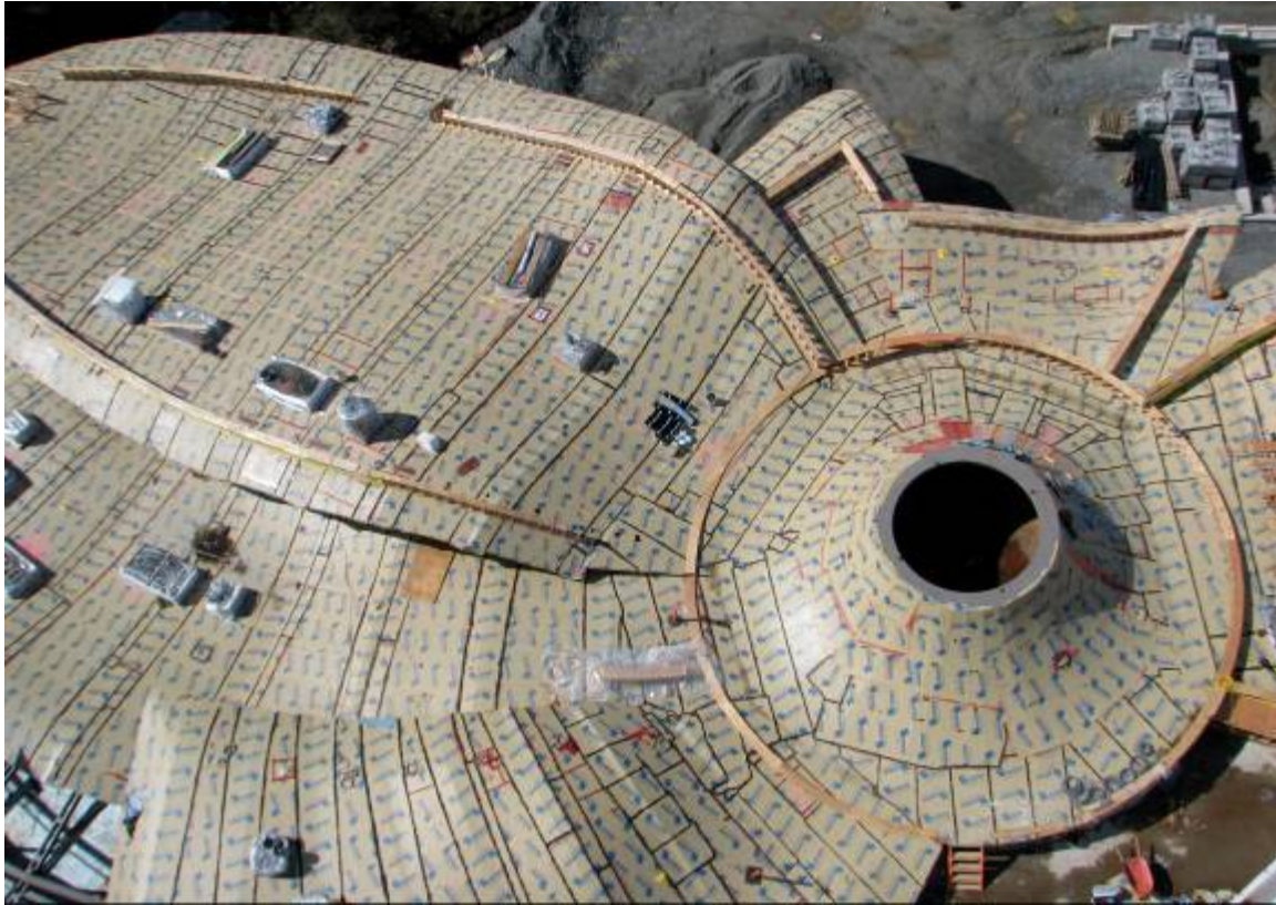
Figure 7 – Aerial view of roof panel erection.
