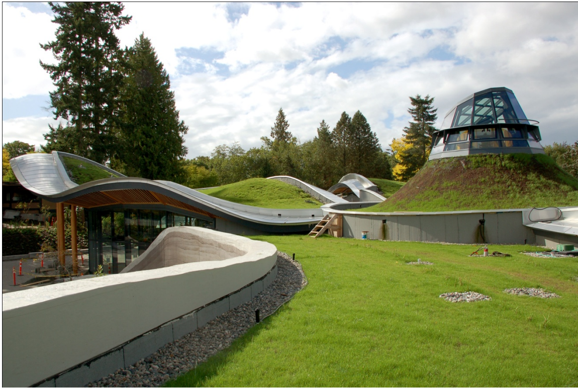
Figure 9 – A model of sustainability, VanDusen features a green roof, rammed earth walls, natural ventilation and is almost solely constructed with timber. Photo credit: Stephan Pasche
