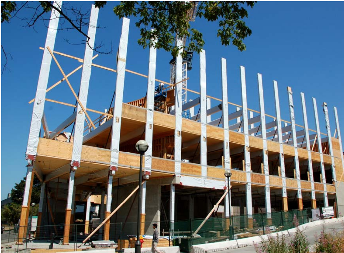
Figure 2 – Crews construct the timber moment frame.
