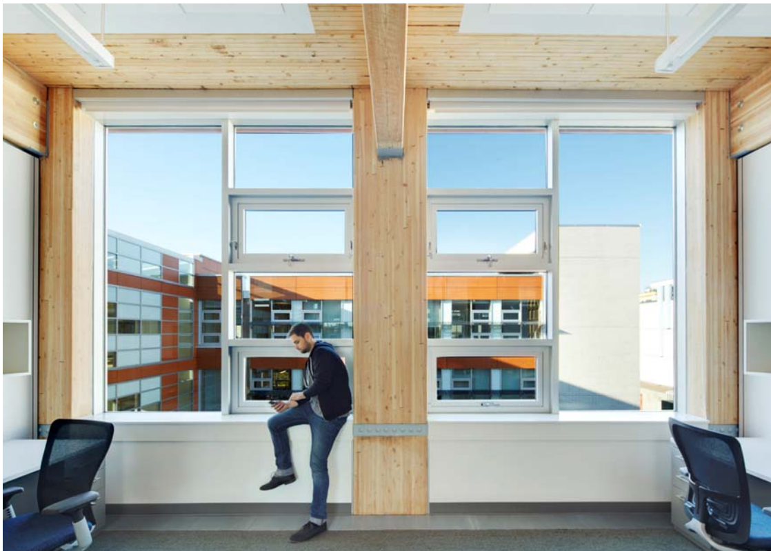
Figure 6 – Moment frame steel strap is exposed on the interior. Credit: Perkins + Will Canada
