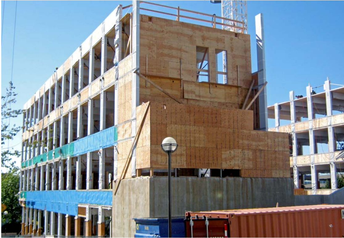
Figure 3 – Completion of moment frame construction.
