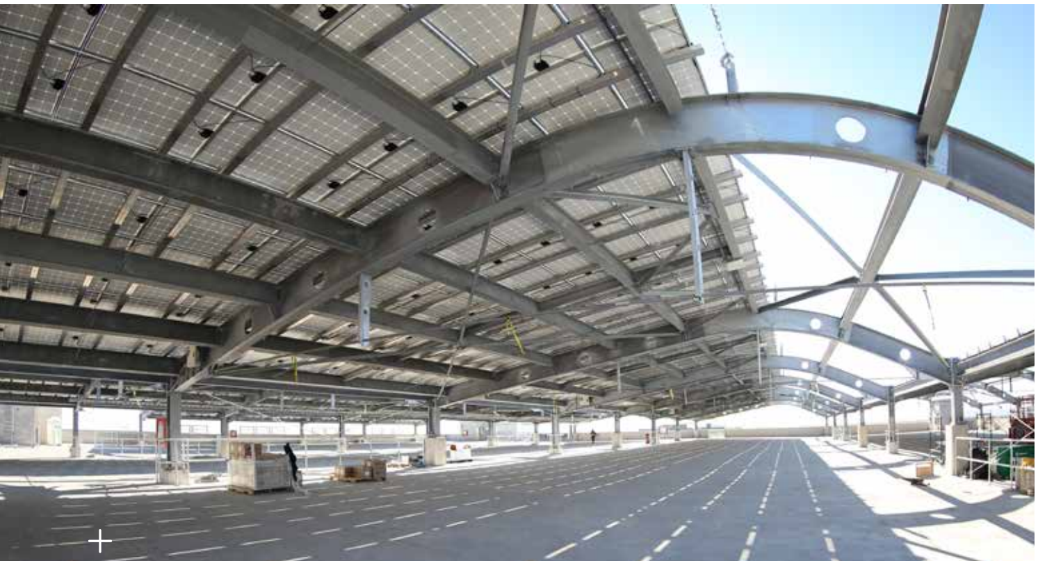
The panel racking structure features a unique design that allows for parking underneath and includes a number of innovations required to meet both the structural and operational requirements of the project without negative impact to the facility.
