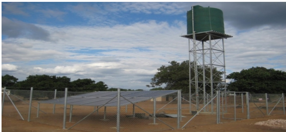
Water reserve and solar panel
