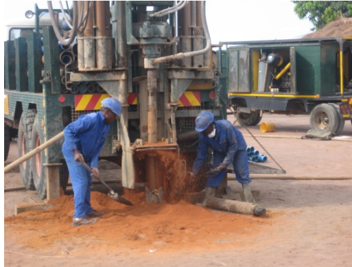
Construction at work
