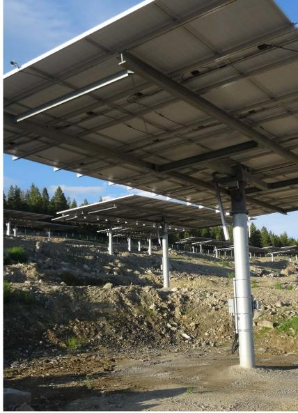
table 12m long X 6m wide on a single 5m support pedestal. There are 4,032 solar panels and hundreds of precisely coordinated power and control cables.
