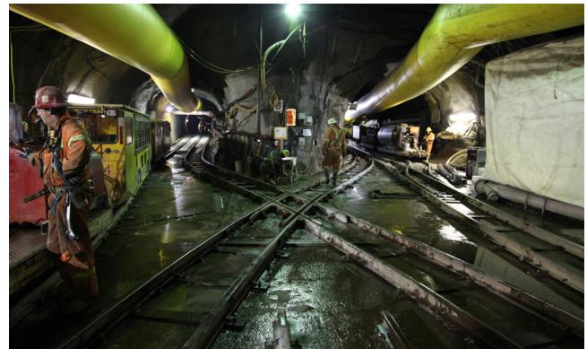
Twin tunnels branching off from the Seymour chamber.
