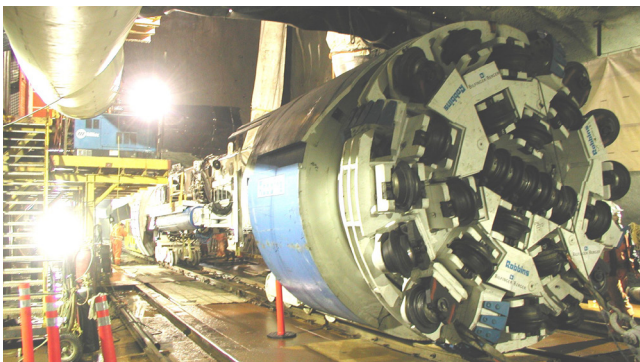
The TBM in Seymour underground chamber as it prepares to drive towards Capilano.
