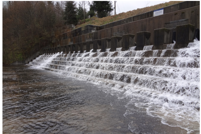
The first treated water to come out of the tunnels on March 12, 2015.
