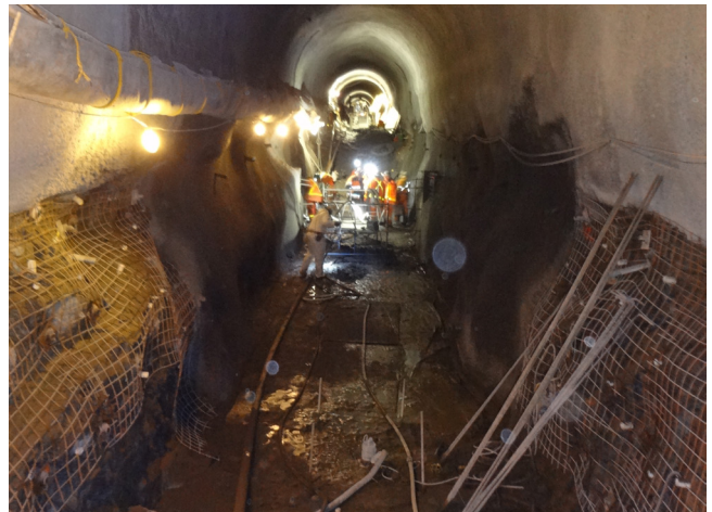
The underground excavation for the treated water rock trap.
