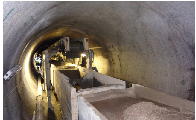
Unlined tunnels in granite bedrock filling muck cars with TBM mined rock to transport out of the tunnel.
