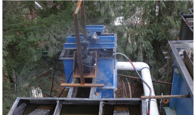
Water treatment plant to treat tunnel construction water before discharging into fish-bearing watercourse.
