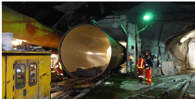
Steel liner beginning its journey into the tunnel.
