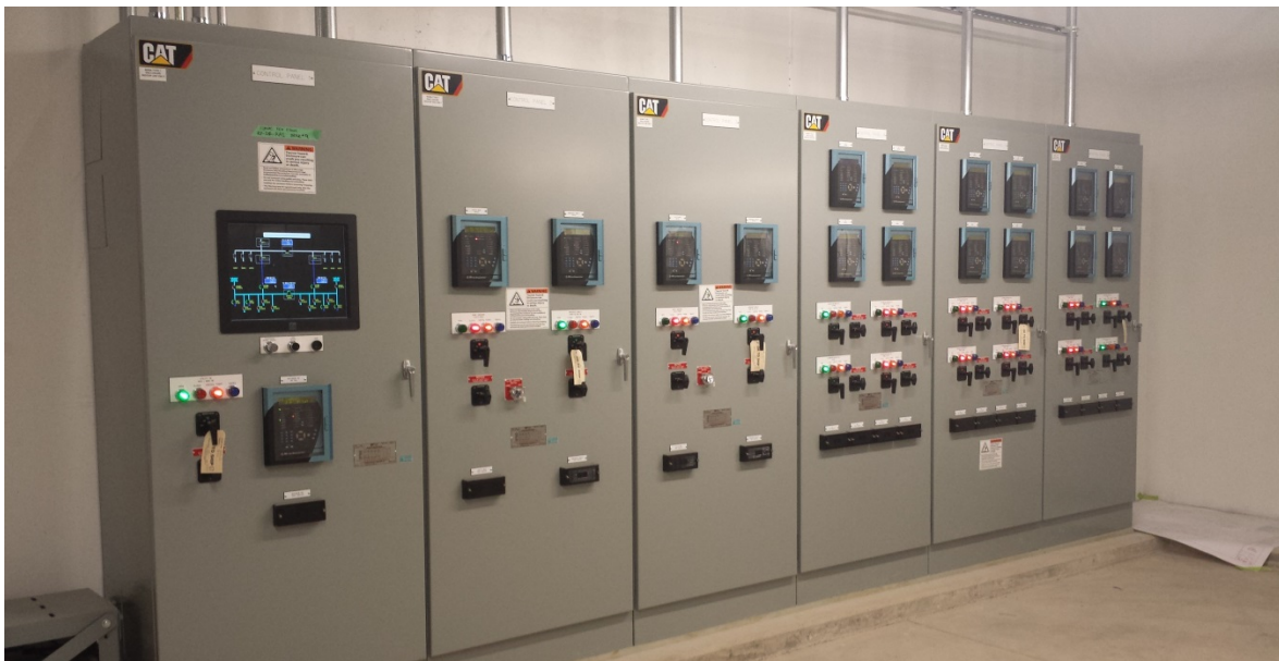
Generator Synchronization Switchboard
