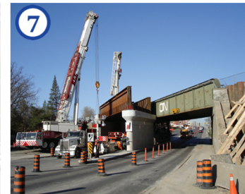
7 Lakeshore East Expansion (New Track)
