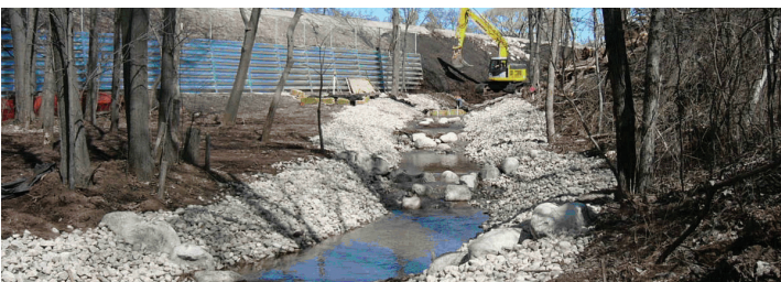
Protective environmental measures during construction
