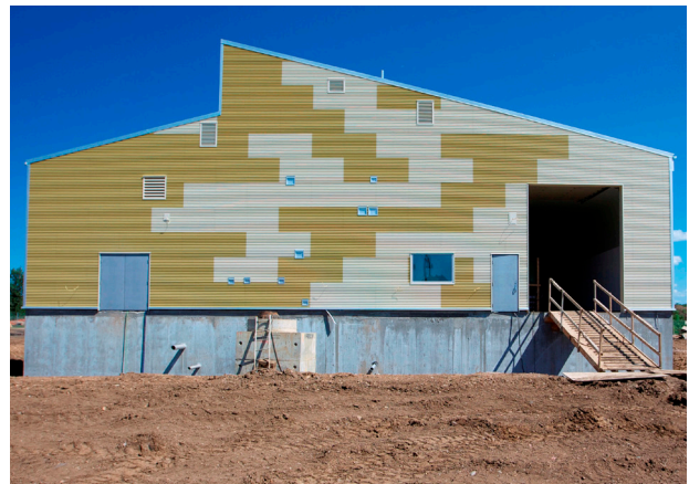
Chateh Water Treatment Plant, June 2010 (in construction)
