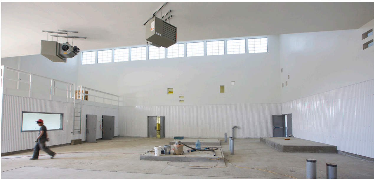
Kalwal “windows” allow natural lighting of the Process Room (in construction in this photo)
