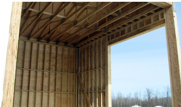
LSL Timber Close up
