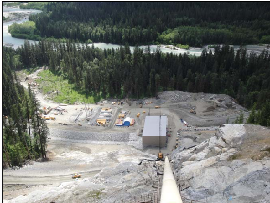
PHOTO 3 – Montrose Powerhouse, Switchyard and Surface Penstock.
