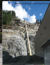
Montrose Pentock and Powerhouse
