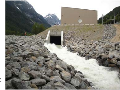
EAST TOBA POWERHOUSE AND TAILRACE
