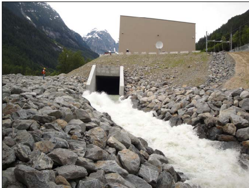
PHOTO 7 – East Toba Powerhouse and Tailrace.
