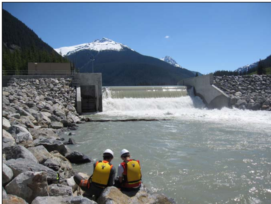
PHOTO 6 – East Toba Intake – Rubber Weir Spillway.
