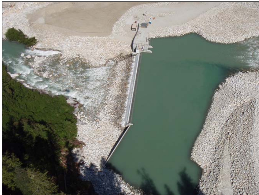
PHOTO 4 – Montrose Intake, Headpond and Avalanche Deflection Berm.
