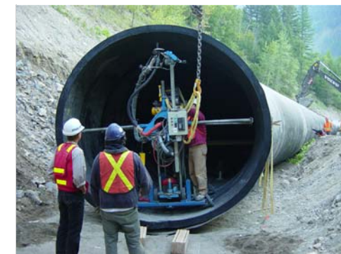
WEHOLITE PIPE WELDING
