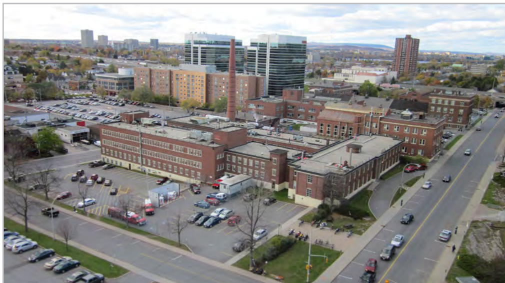
Central and Northwest Quadrants before remediation
