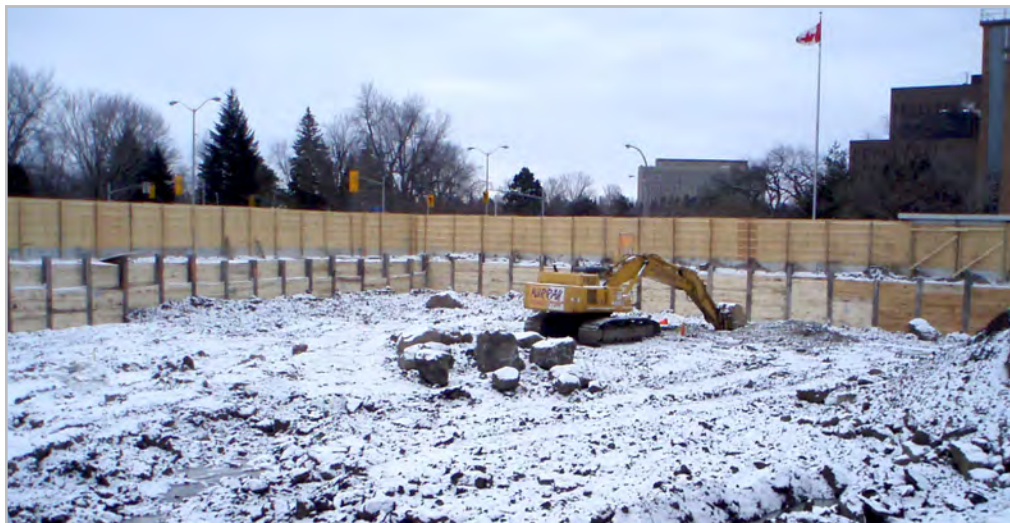
Excavating through frozen ground in the Southeast Quadrant
