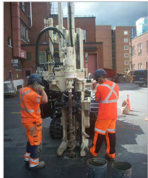
Drilling a borehole using a solid stem auger drill rig
