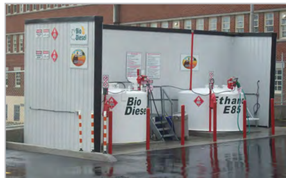
Reinstated vehicle fuel tanks in Central Quadrant
