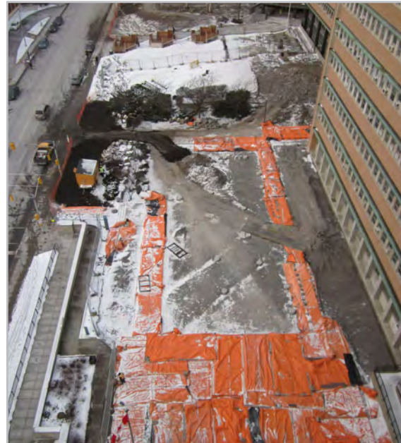
Protection of exposed features and concrete from freezing during the remediation of the front of 601-615 Booth St in the Southeast Quadrant
