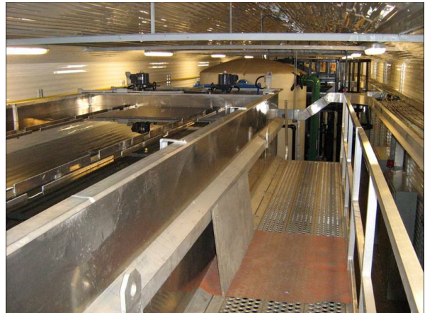
Treatment Plant Interior
