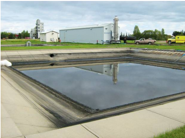
Contaminated Water Pond
