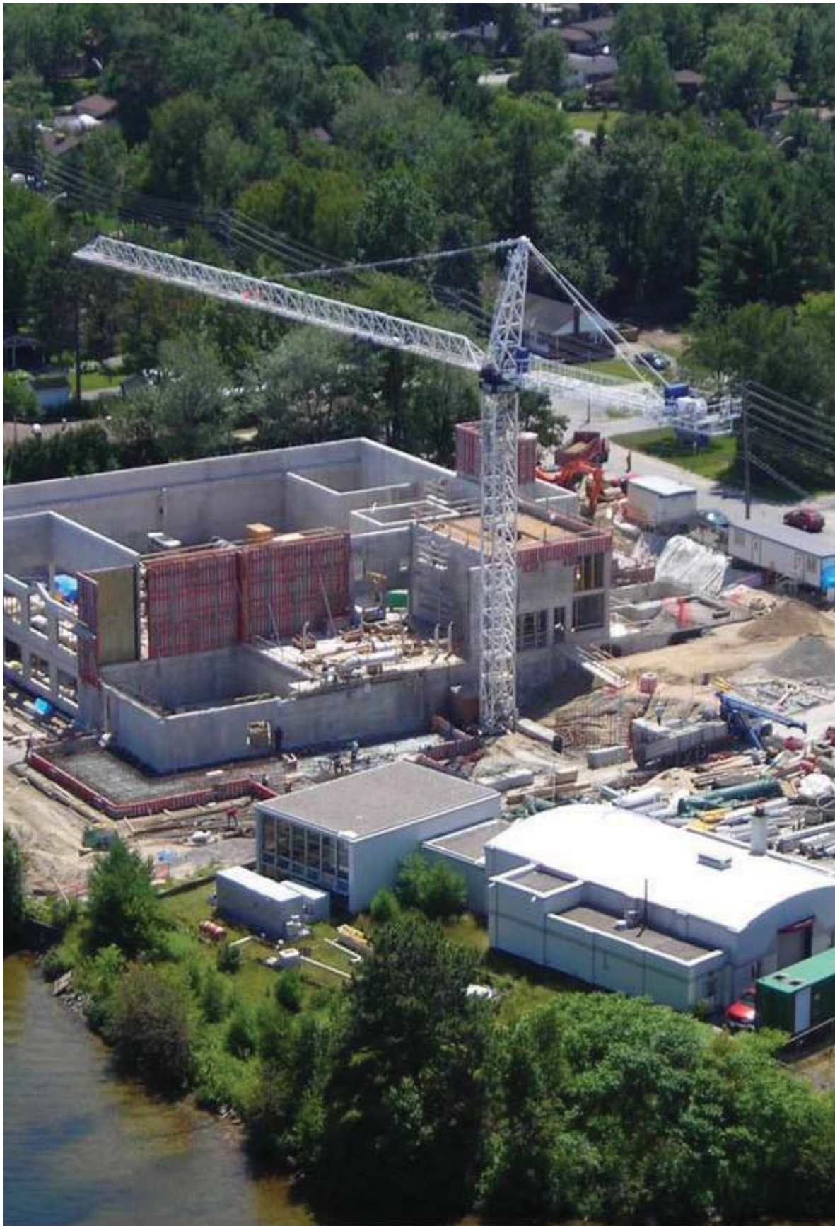
The North Bay Water Treatment Plant is the largest dual-membrane, high recovery plant in North America achieving >99% recovery of the source water.
