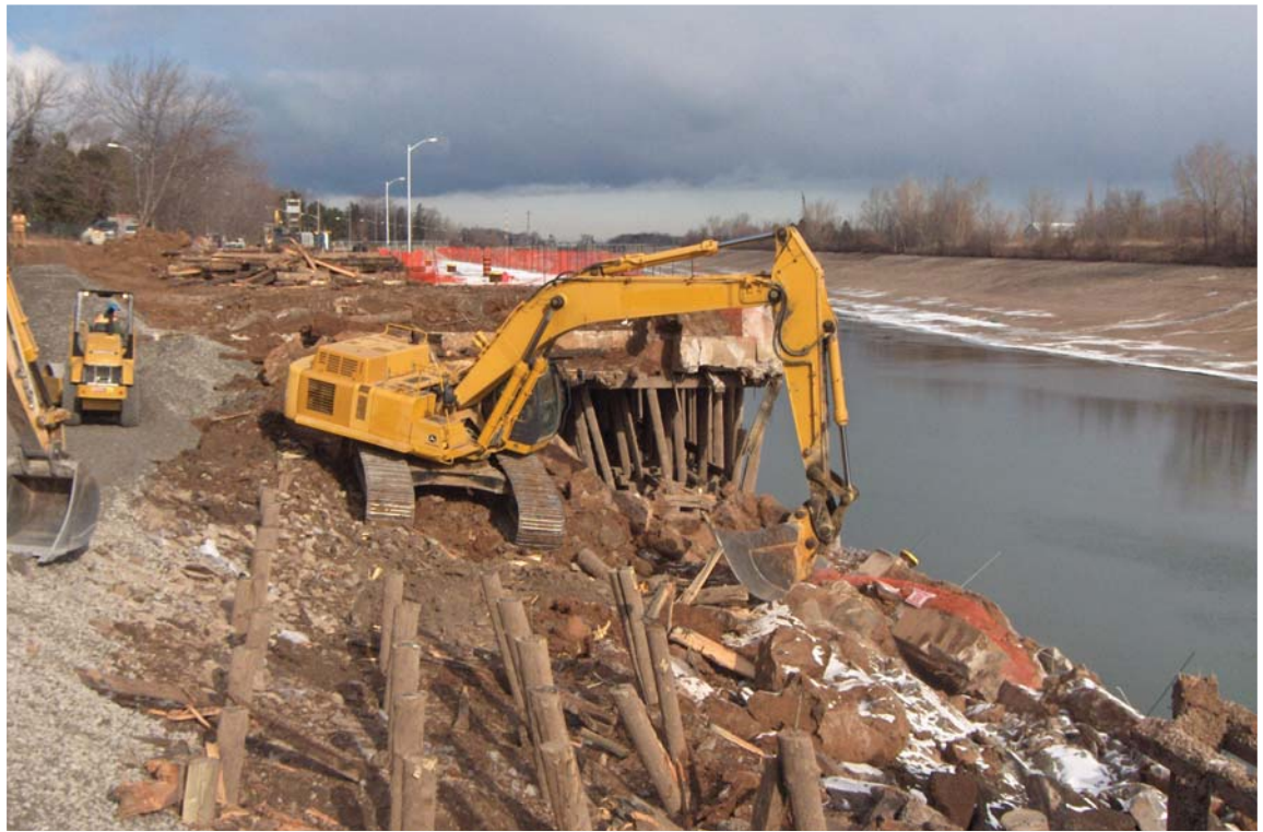
Photo 3 • Removal of debris
