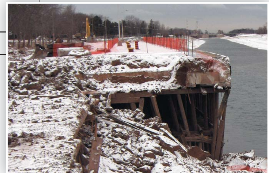
Photo 5 • View of collapsed deck
