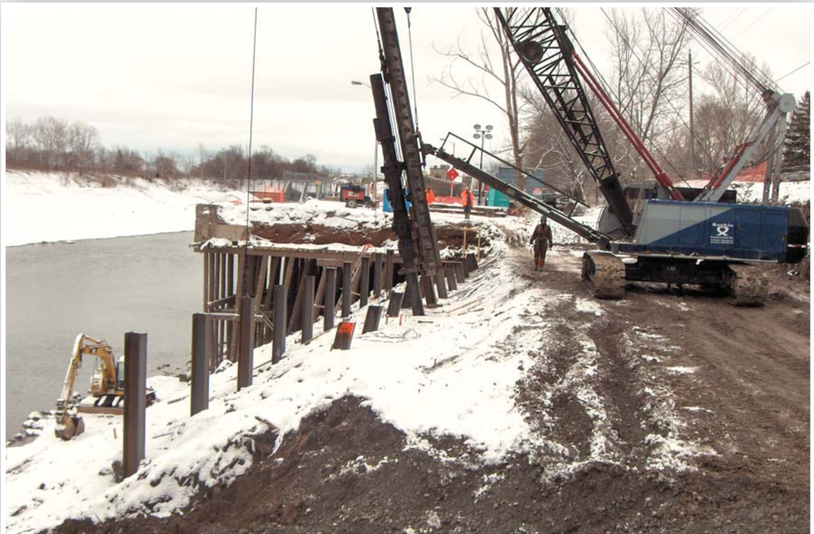
Photo 4 • Steel H pile installation
