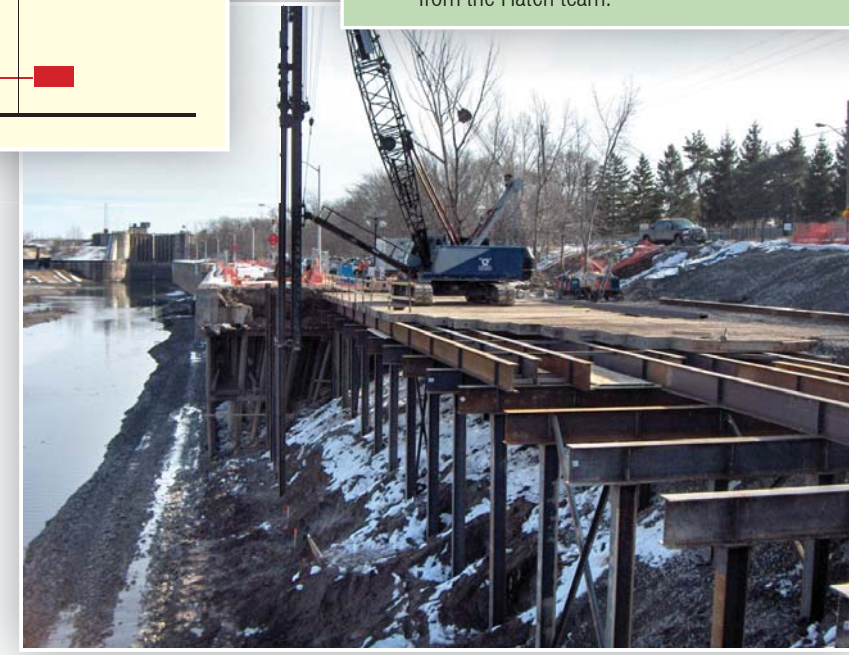
Photo 6 • Pile driving (note rig on top of new deck)
