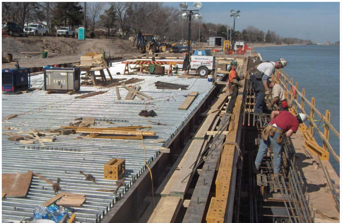
Photo 8 • Deck nearing completion
