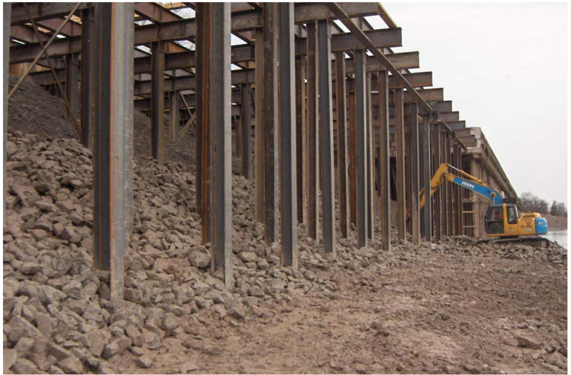
Photo 7 • Canal view of new H piles, beams, girders and placement of slope protection material
