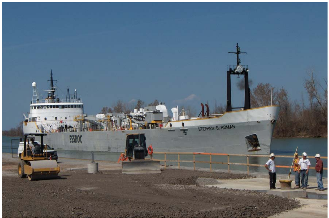
Photo 9 • Granular fill placement on reconstructed tie-up wall as ship passes through canal
