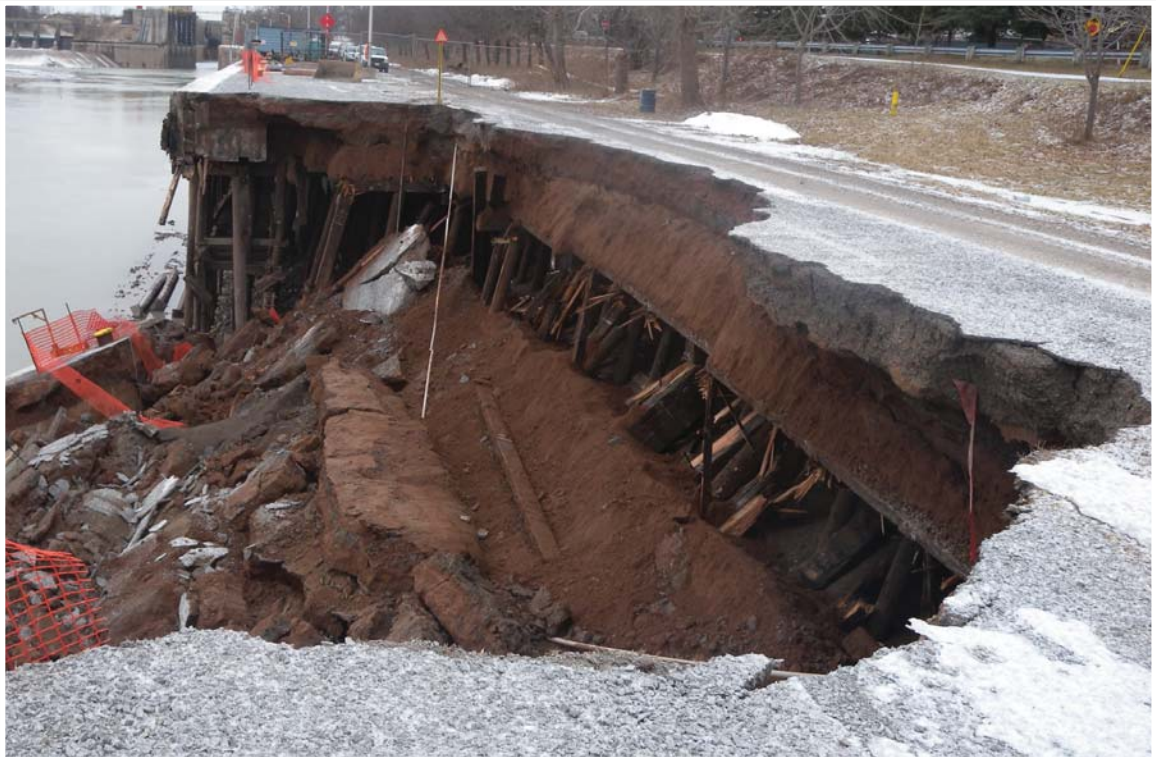
Photo 2 • View of collapsed section (January 26, 2010)
