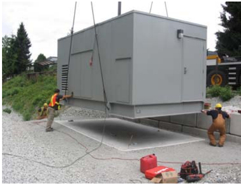
Installing one of two new 500-V substations
