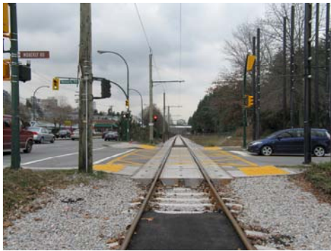
Vancouver's first road crossing by a light rail vehicle that relies on traffic lights without gates or other railway signals
