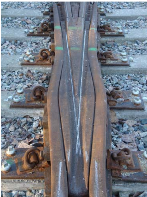
Modern, flange-bearing frogs smooth turnout transitions
