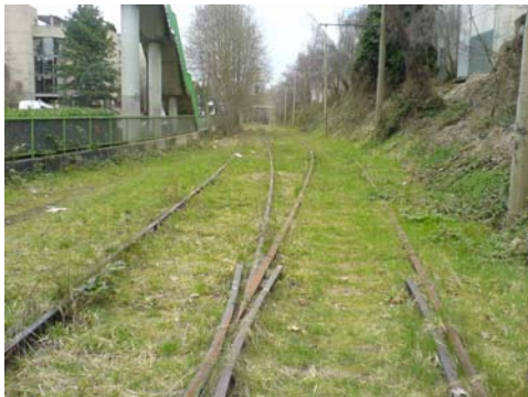
The rail corridor to Granville Island was dilapidated and unsuitable for modern streetcar use at the start of the project
