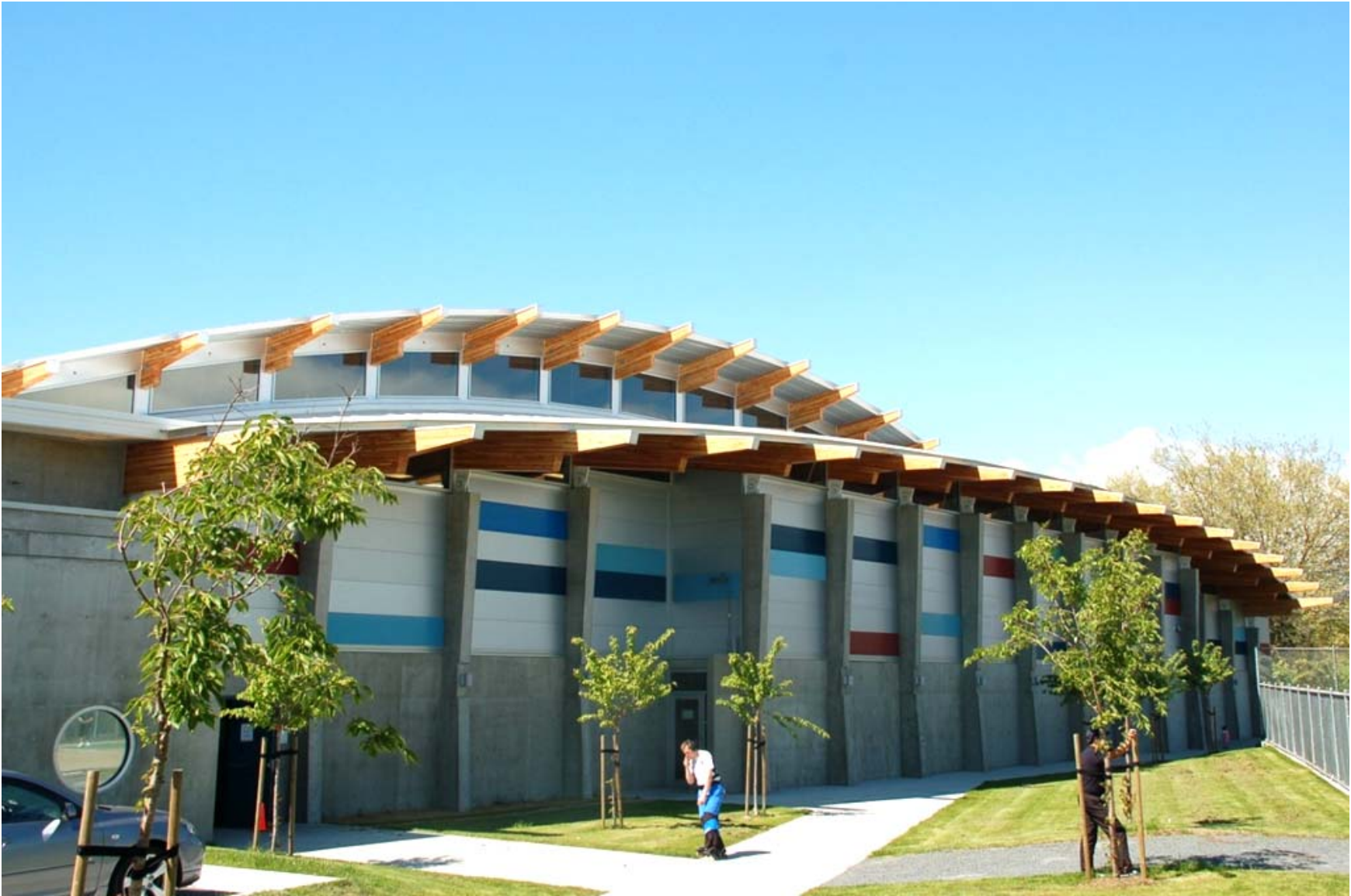
Exterior view of east side.
