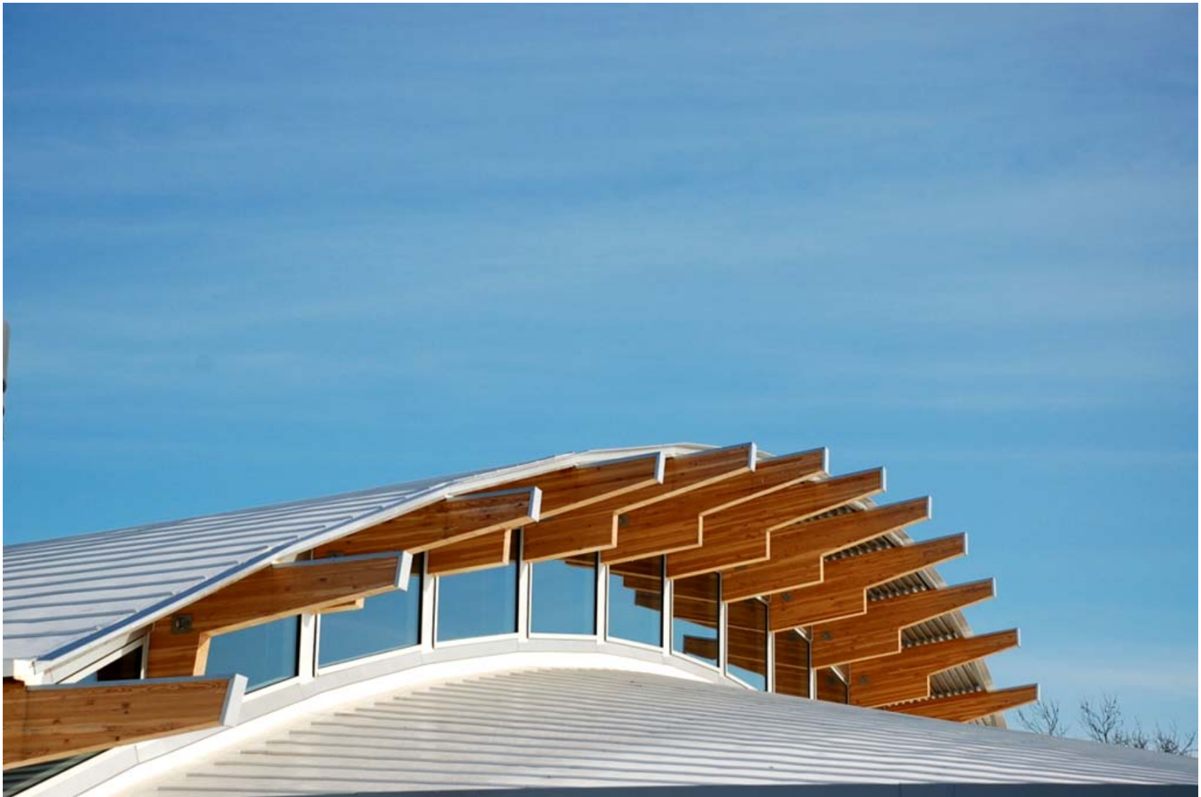
Exterior view north-west – clerestory detail.
