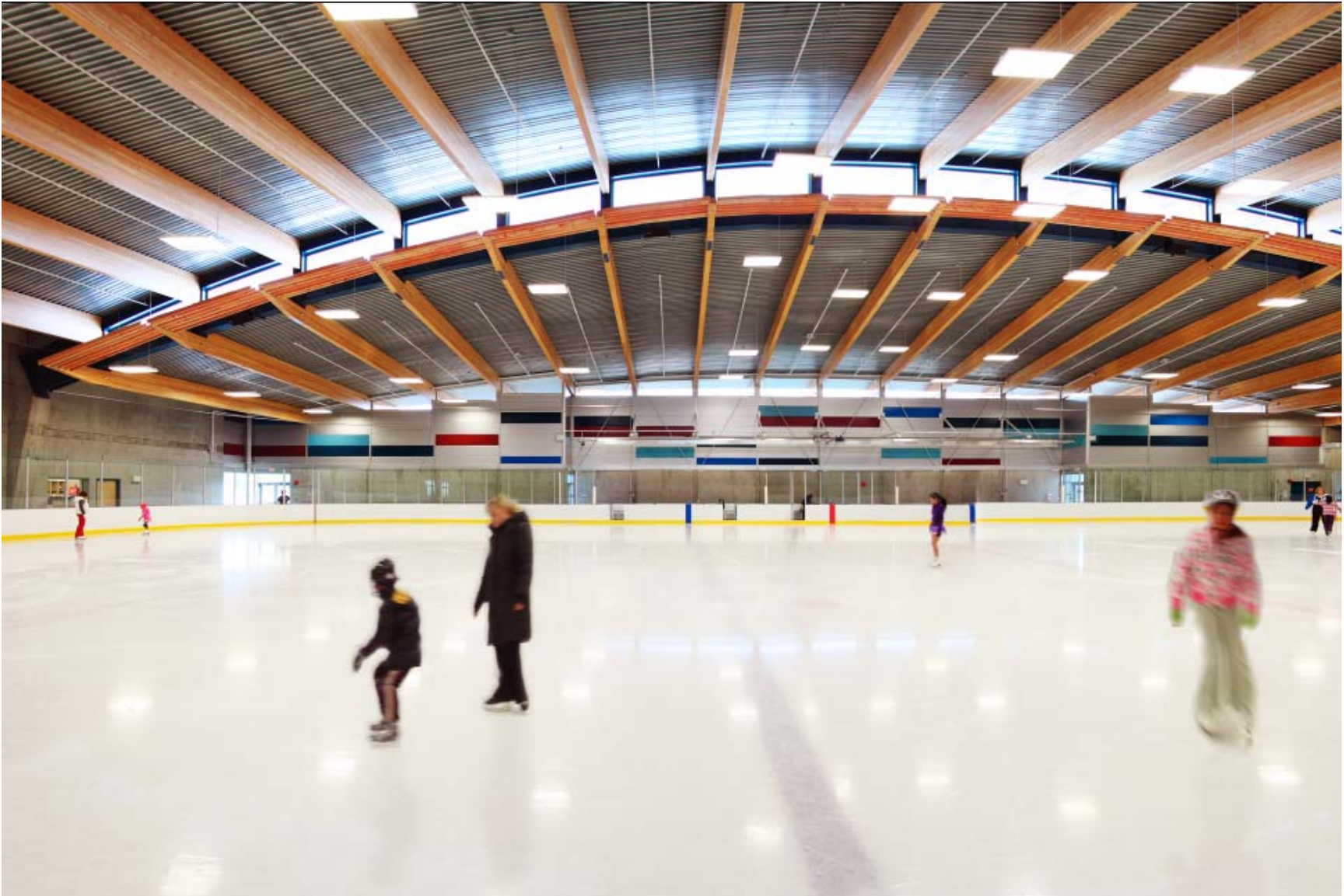
Interior view east.
