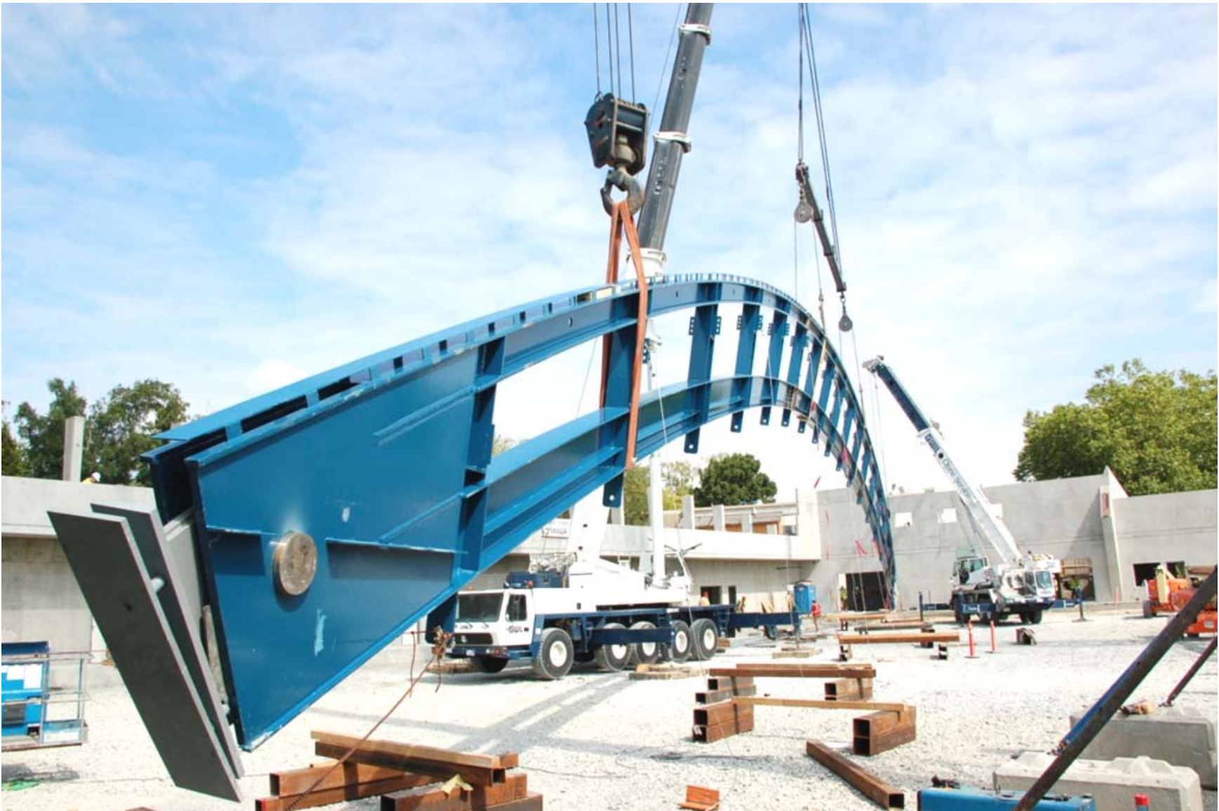
Vierendeel Truss Arch – Construction.
