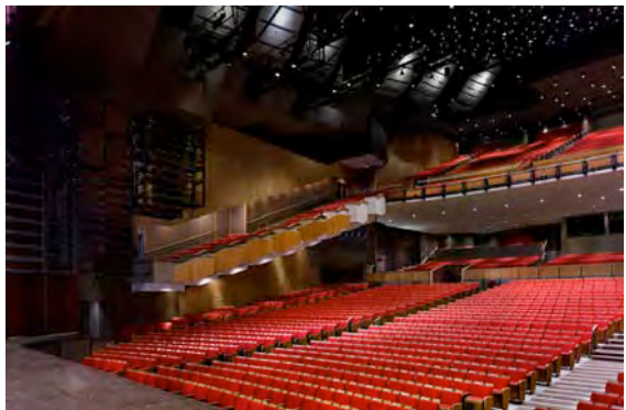
Figure 2 View of the renovated Queen Elizabeth Theatre from the stage. Lateral reflectors can be seen in the ceiling and on the face of the side balcony.
