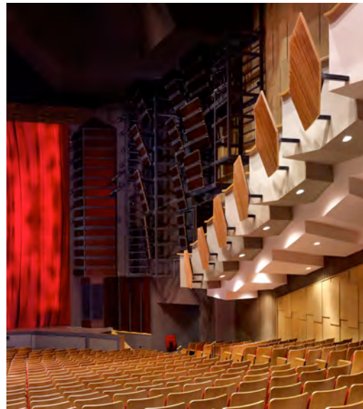
Figure 6. Zone 2 balcony fascia reflectors are seen in the foreground. Note how they progressively move toward the centre-line of the room.
