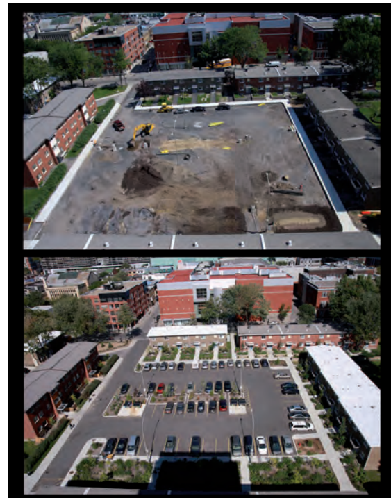
Aerial photo - During and after rehabilitation
