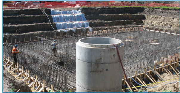
A sump system employed during construction for dewatering.
