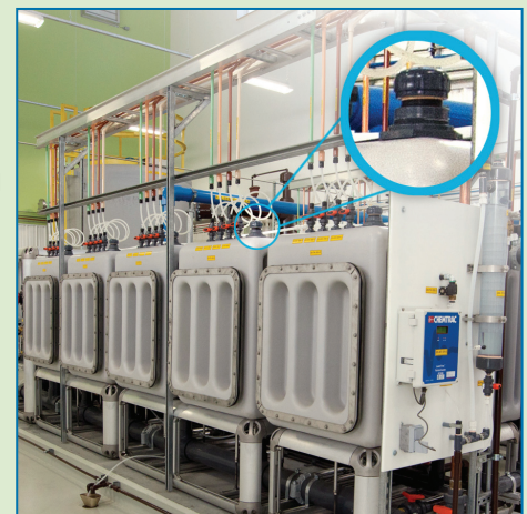
Chemical fill ports with easy screw-on cap.
