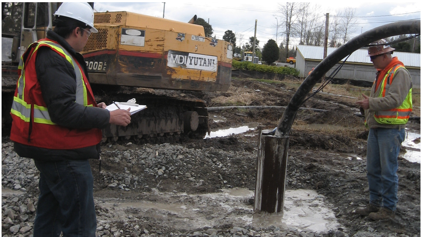
Grout placement in the 50-m-deep grouting trial hole in progress.
