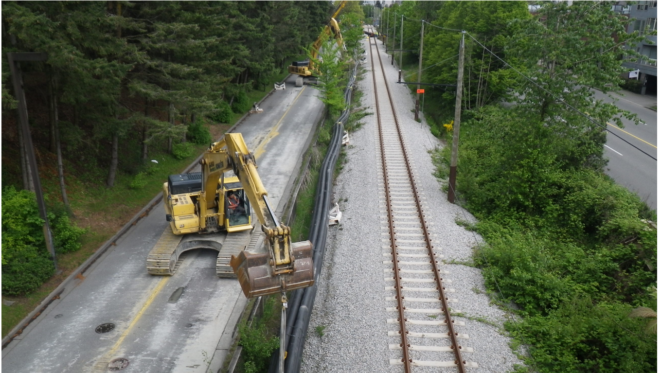
Conduit Bundle Fusing and Temporary Laydown Area in Heritage Railway Corridor
