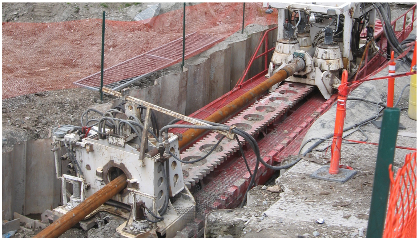
HDD Drill Rig at David Lam Park
