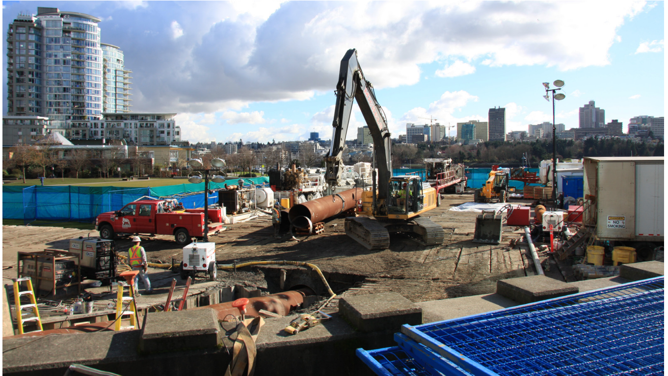
David Lam Park Drill Entry Work Area
