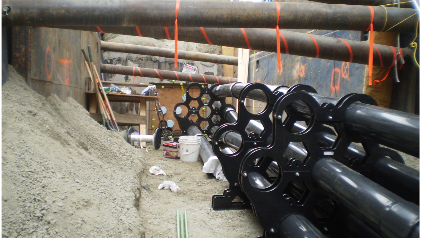
Duct Bank Construction at Laurel Street Transition Tie-in to Manhole
