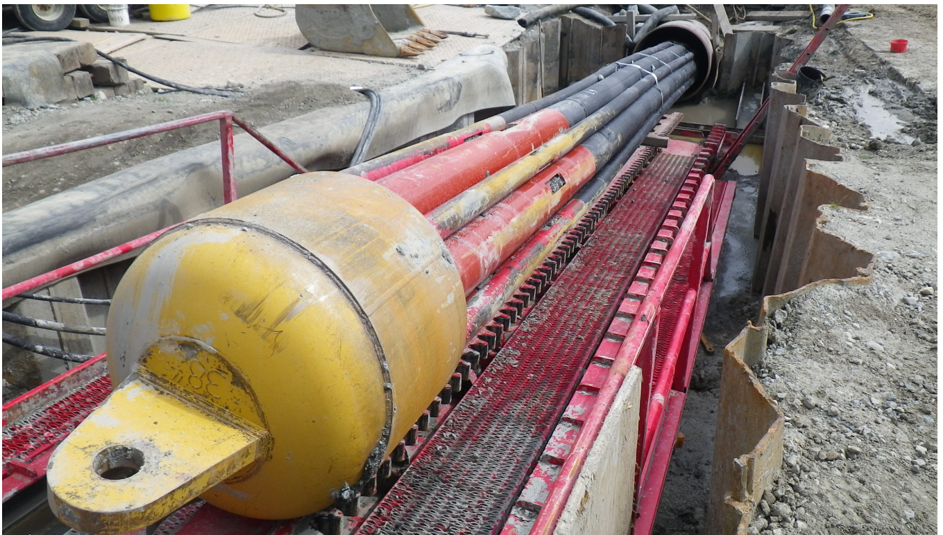
Pull Head at Drill Exit after Successful Pullback
