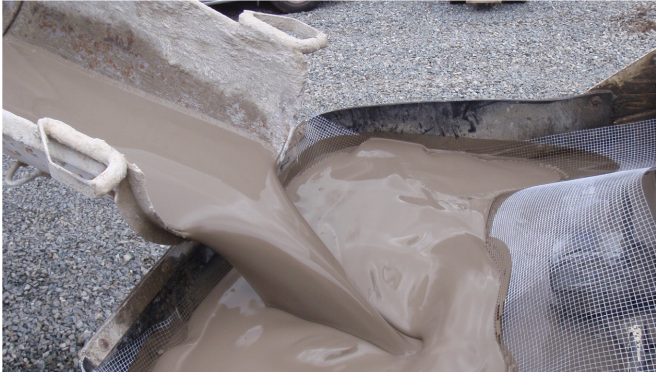
Batching of Thermal Grout for Pre-Production Field Trial
