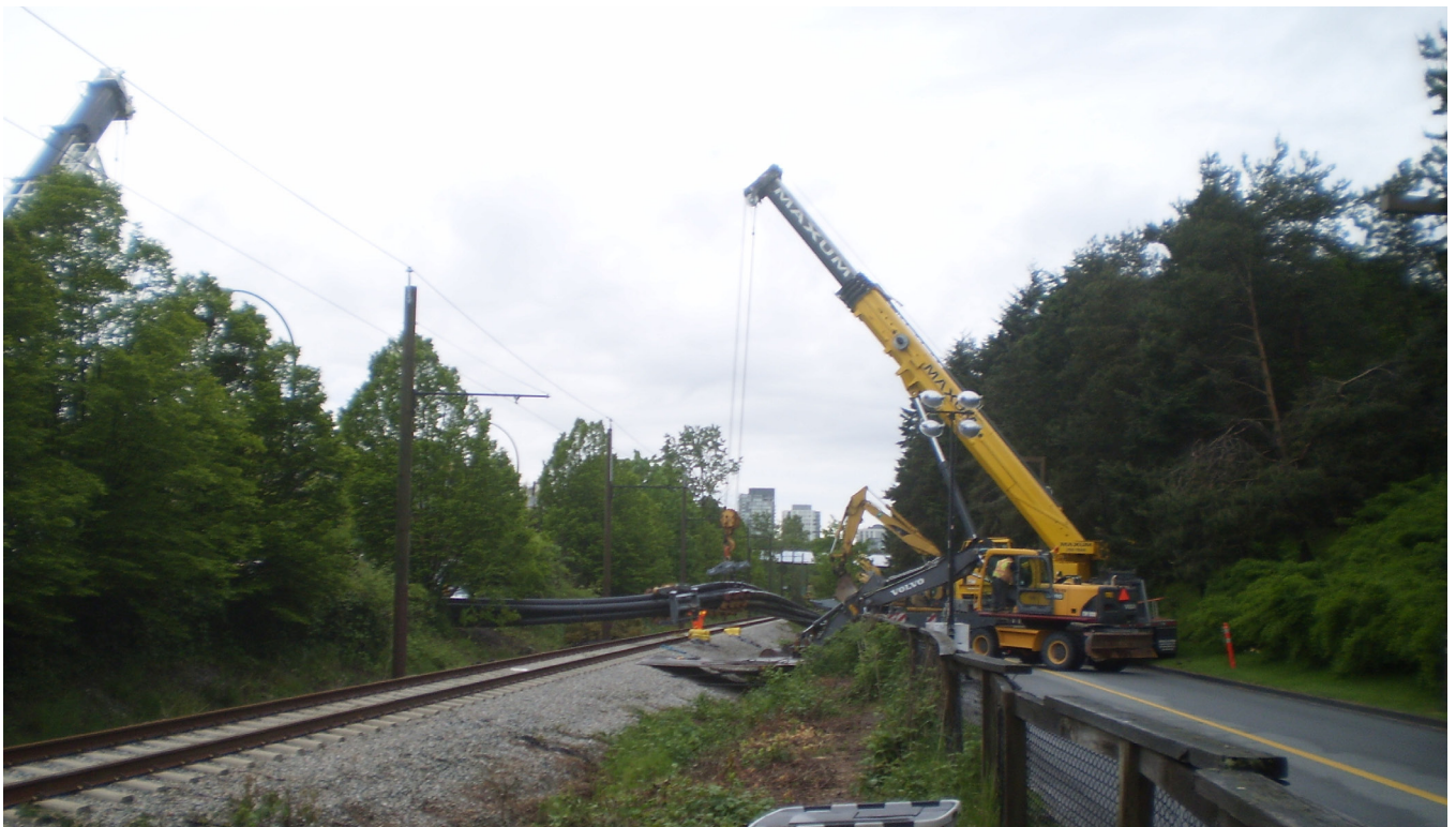
Duct bundle transported from Railway Heritage Corridor to the Pipe Laydown area in downtown Vancouver.
