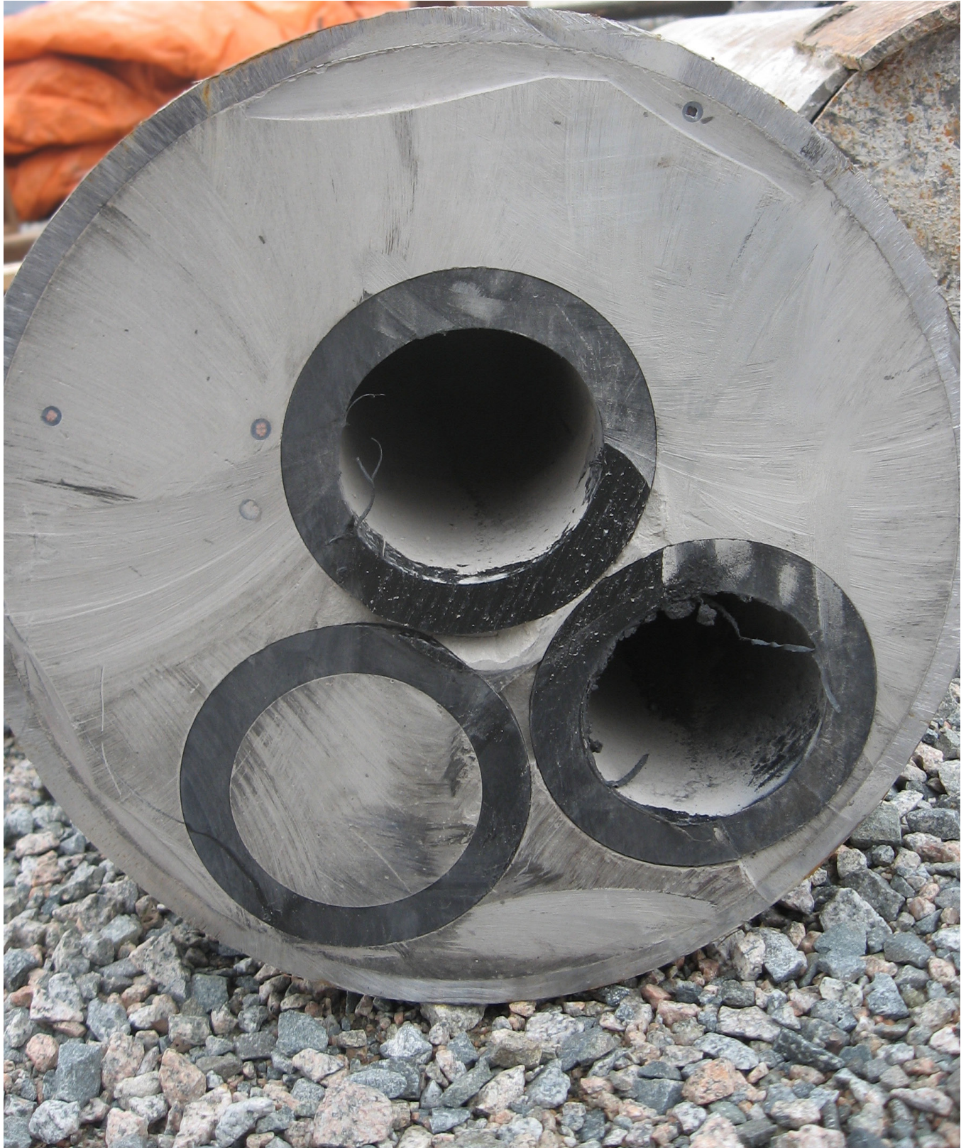
Grout trial showing a cross section of the grout surrounding the trial pipe bundle.
