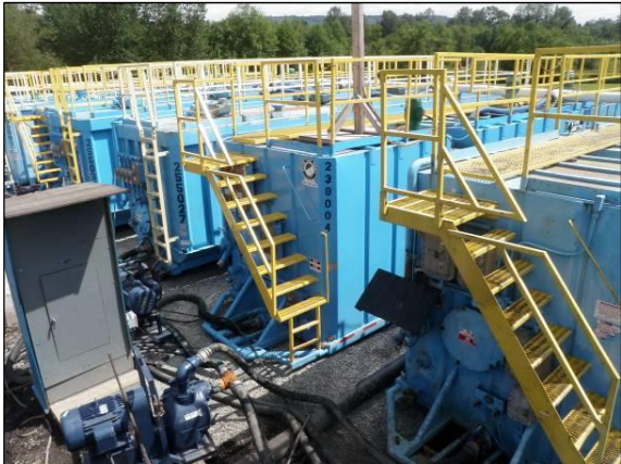
Equilization Tanks at the Treatment Plant
