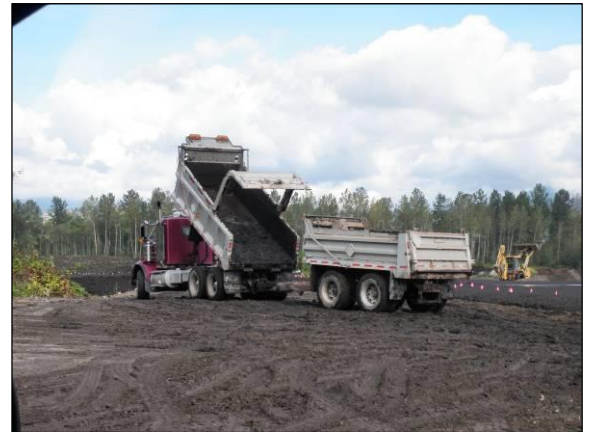
Trucks Loading and Hauling Away Sediment
