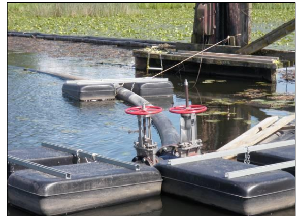
Lake Pipeline in Use
