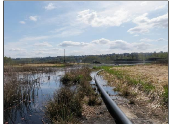
Land Pipeline Transporting Dredgeate to the Upland Treatment Plant
