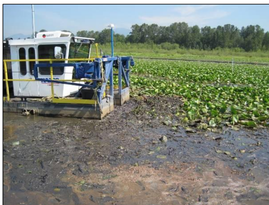
Hydraulic Suction Dredge Cutting Through Shallow Water & Heavy Vegetation
