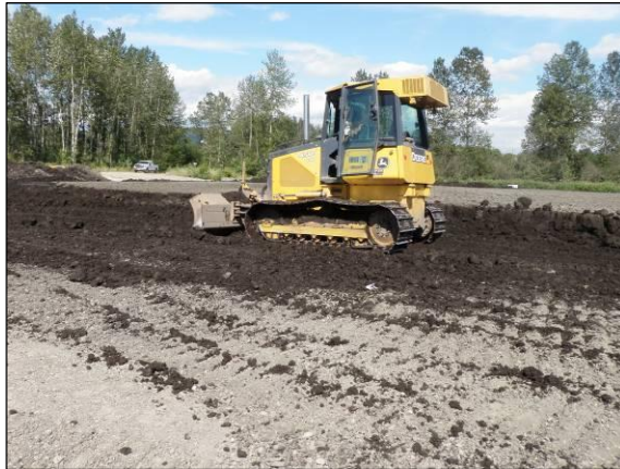
Spreading/Grading of Sediment as Subgrade
