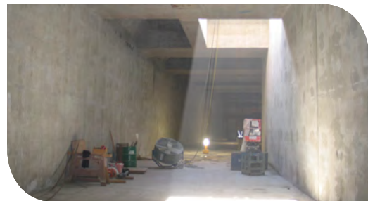
Inside northbound tunnel at mechanical opening
