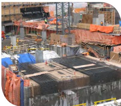
Roof Reinforcement and Transfer Girders Between Gridlines 9 and 12 January 2009
