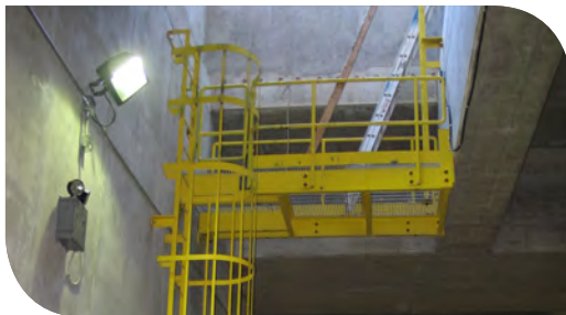
Temporary access to tunnel Cavity
