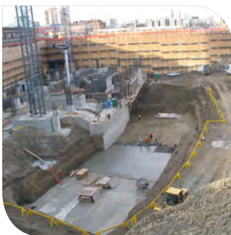
Placing Mudslab for LRT, October 2008
