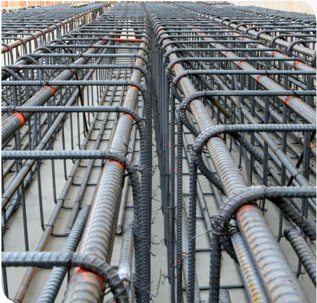
Base Slab Reinforcement
