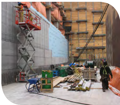
Southbound Looking West January 2009
