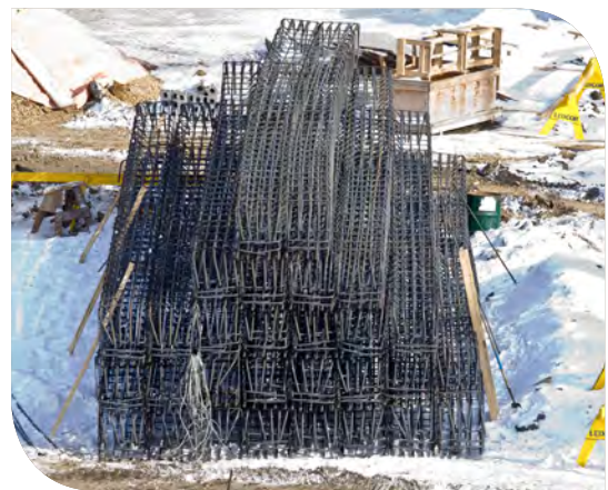
Stockpiled Reinforcing Cages
