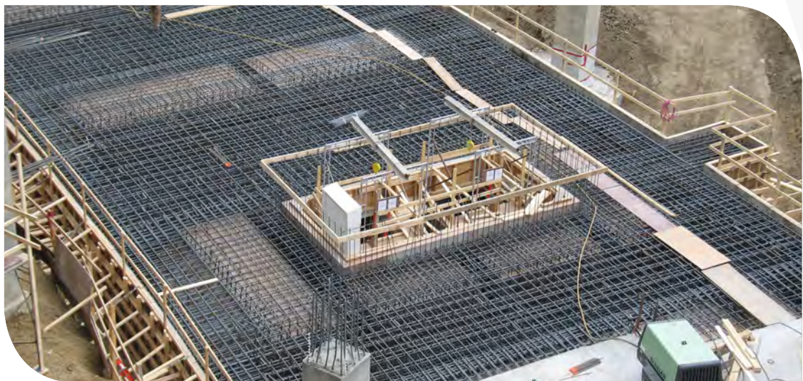
Completion of Tunnel Roof May 2010
