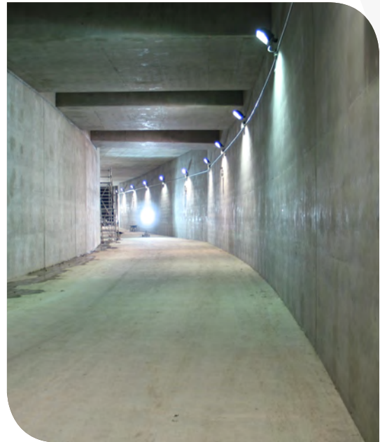
Temporary Lighting in Southbound Tunnel
