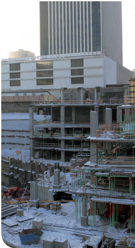
Complex coordination of construction east of gridline 14; CN Tower in background
