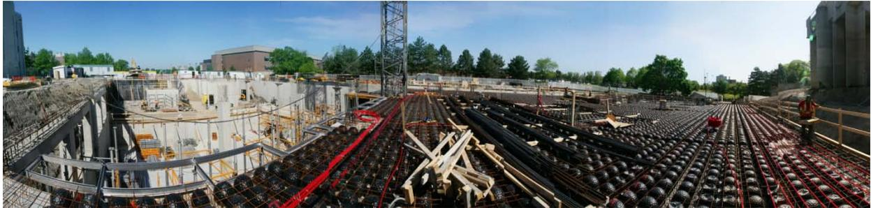
When we began the project, our schematic design identified reinforced concrete as the best option in terms of its ability to provide a robust and economical structure. Concrete was also adopted for aesthetic reasons, with the architect choosing to express architectural concrete columns and slab soffits around the day-lit perimeter of the building.
